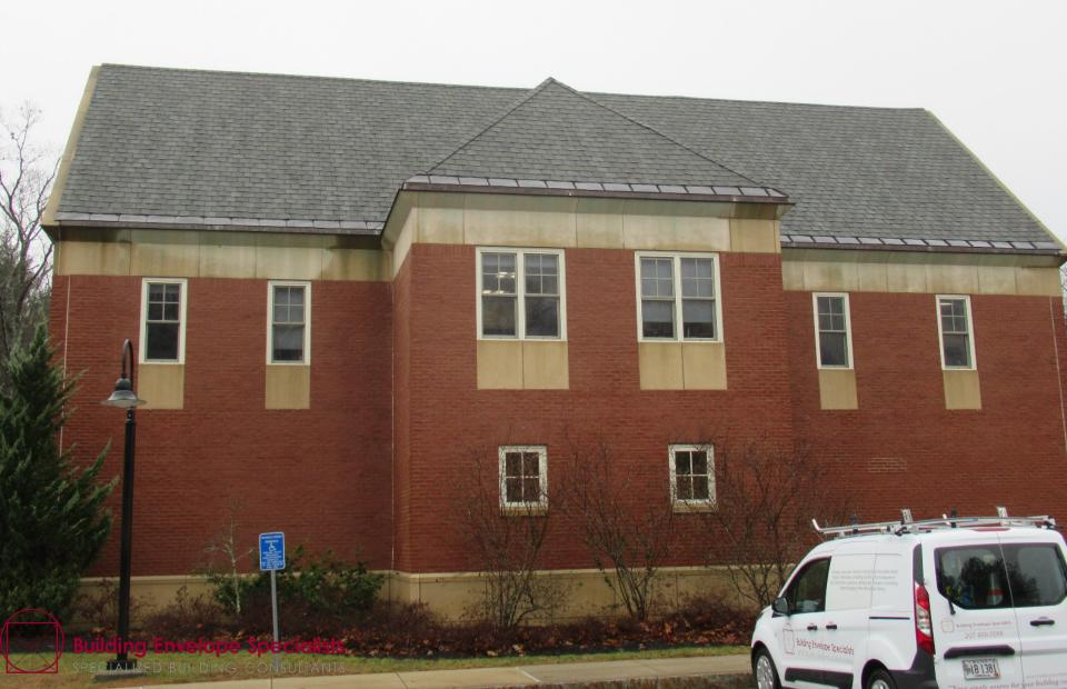
North elevation has had some repairs that have mitigated some of the moisture problems. Note, precast has been discolored.
