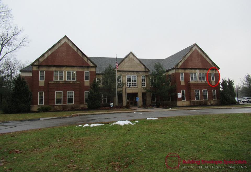
East elevation has the least moisture problems. Note that the corners have significant roof runoff. Add gutters?
