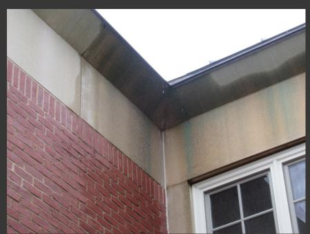
Walls at roof valleys are receiving significant runoff water during rain events.
