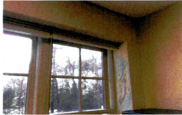
Figure 2: Water infiltration resulted in blistered paint on the window header and jamb in Room 224.
