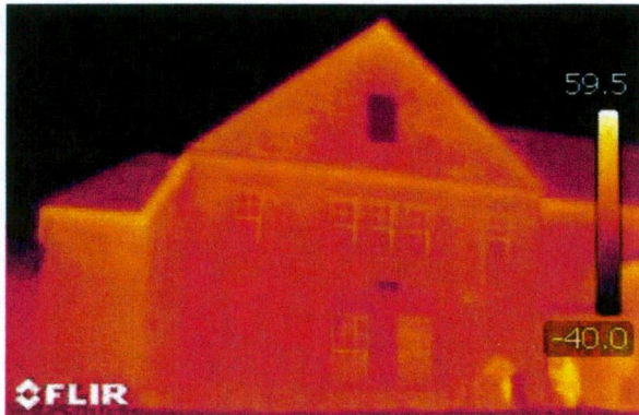
Figure 9: Exterior thermographic image shows warm air exfiltration at multiple exterior wall locations.
