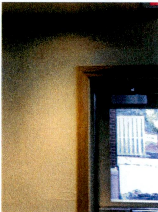
Figure 11: Water infiltration resulted in blistered paint on adjacent to the door in the Assembly Room
