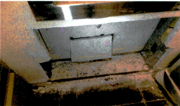
Figure 3: Evidence of water infiltration based on rusted metal-stud framing inside the Payment Drop closet on the 1 st floor
