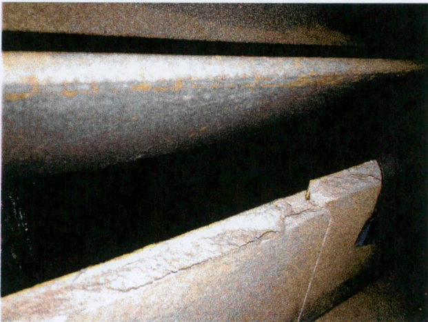
Figure 19: View of the roofing underlayment that is not supported at the roof to wall transition.
