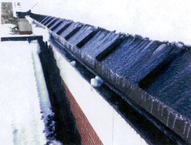
Figure 10: Precast stone shelves are located at the eave locations allowing snow, ice, and water to build up. Eave locations were covered with a sheet metal cap.
