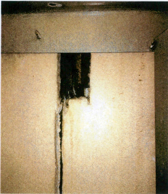
Figure 18: DensGold cut to allow steel anchor for precast.
