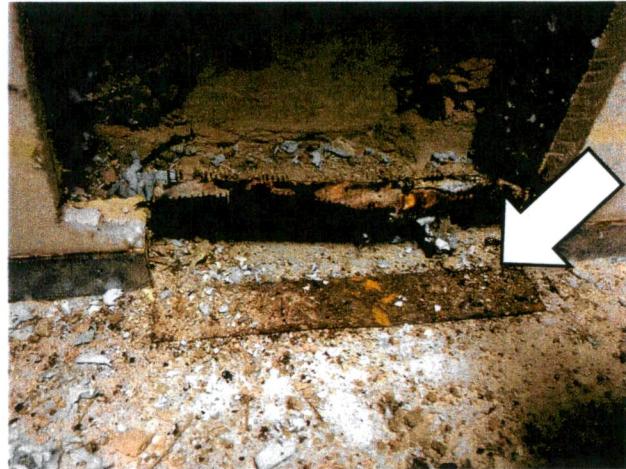
Figure 23: The bottom track of the metal stud was observed to be corroded at interior test cut locations.
