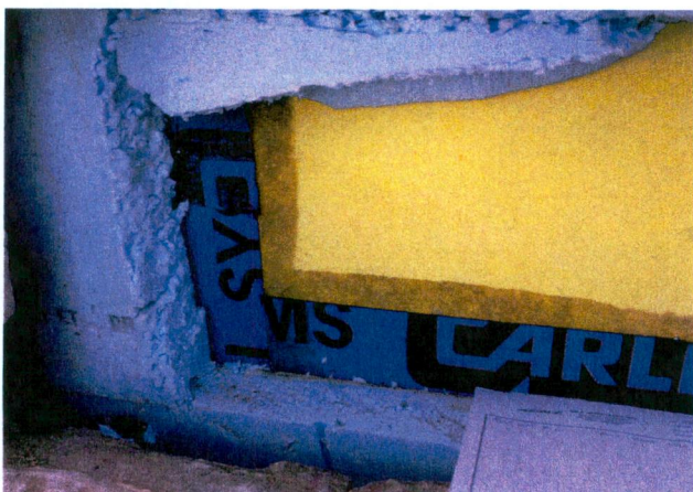
Figure 16: The DensGlass Gold sheathing seams appear to be stripped in with AVB transition membrane.
