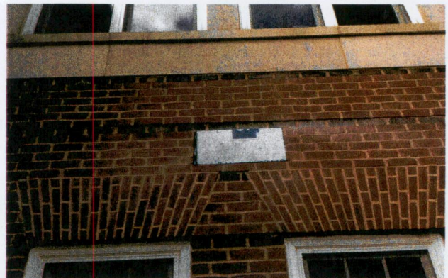
Figure 12: Jack arches are installed above the first-floor windows.
