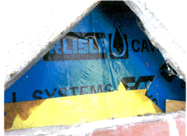
Figure 17: SA membrane was observed to have multiple fish mouths and wrinkles.
