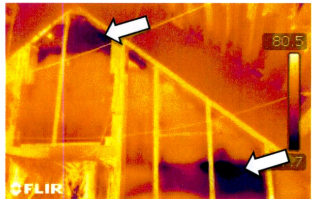
Figure 5: Thermographic image from inside the attic shows cold air infiltration at the gable wall transition to the roof ridge.
