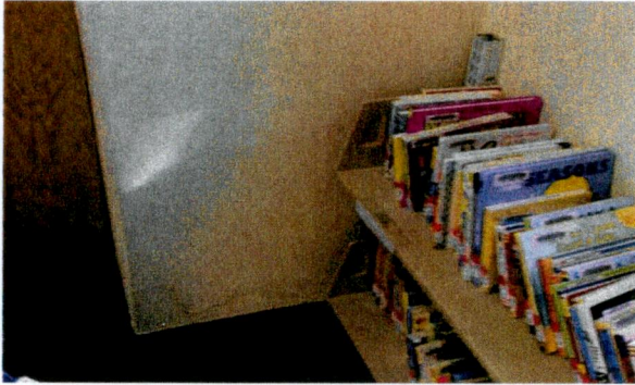
Figure 10: Water infiltration resulted in blistered paint on the interior wall in the Children's Library.
