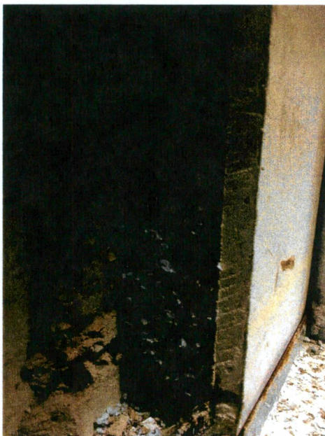
Figure 6: View of the typical wall construction from the interior with precast concrete exterior cladding.
