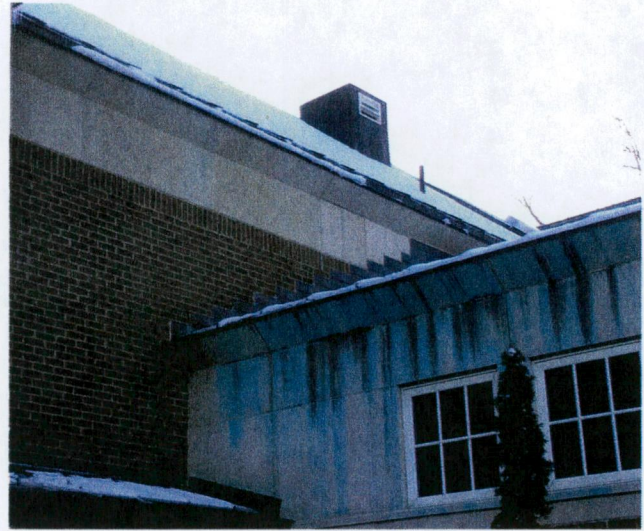
Figure 13: Heavy copper staining on the precast was observed along the assembly room walls.
