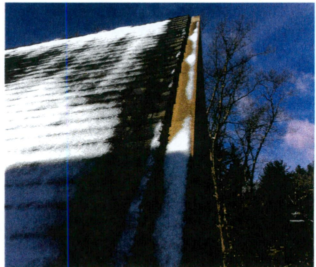
Figure 8: Exposed precast extends out beyond the roof edge on the rake edges of the roof.
