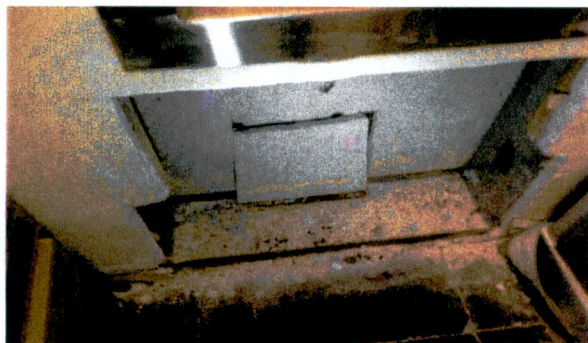
Figure 6: Evidence of water infiltration based on rusted metal-stud framing inside the Payment Drop closet on the 1 st floor
