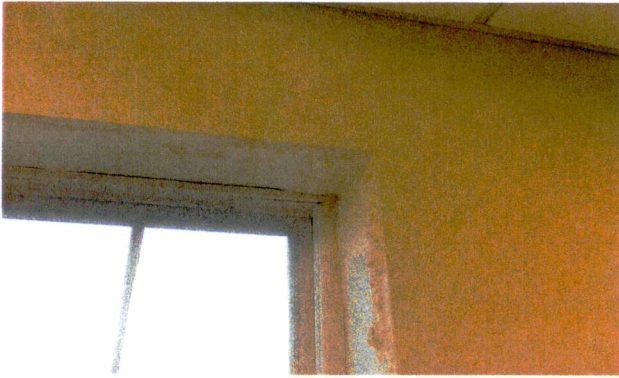
Figure 2: Blistered paint on the window header and jambs was observed at multiple locations.
