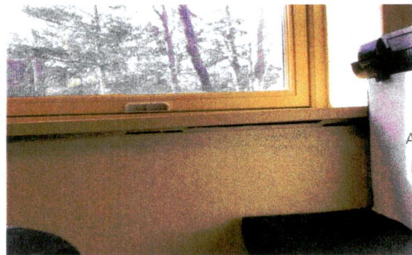
Figure 3: Bowed/displaced interior stool in Room 227.
