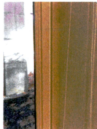
Figure 8: Blistered paint on interior wood trim adjacent to a window.
