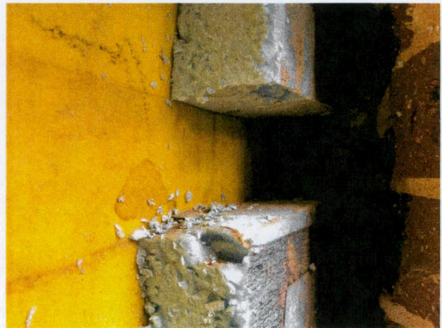
Figure 14: Gaps in the insulation were observed at multiple locations.
