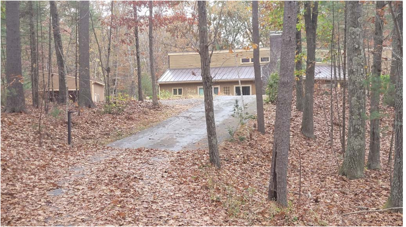
20 Rowley Rd Boxford, New Barn – Street View (north/north west)
