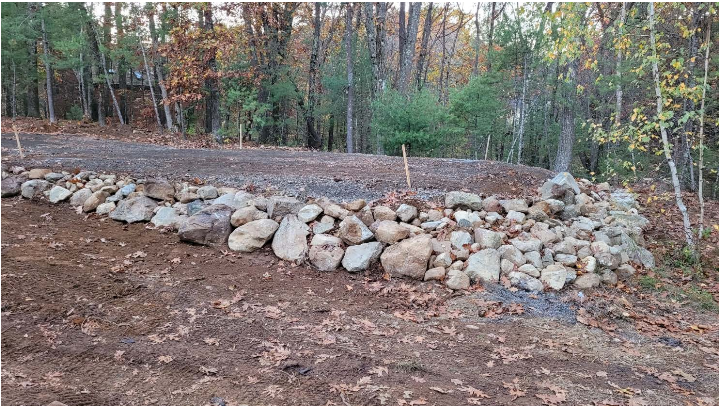
20 Rowley Rd Boxford, New barn Location – Side View (west)
