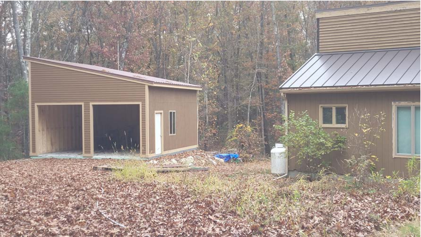
20 Rowley Rd Boxford, New Barn – front view from existing driveway (north)
