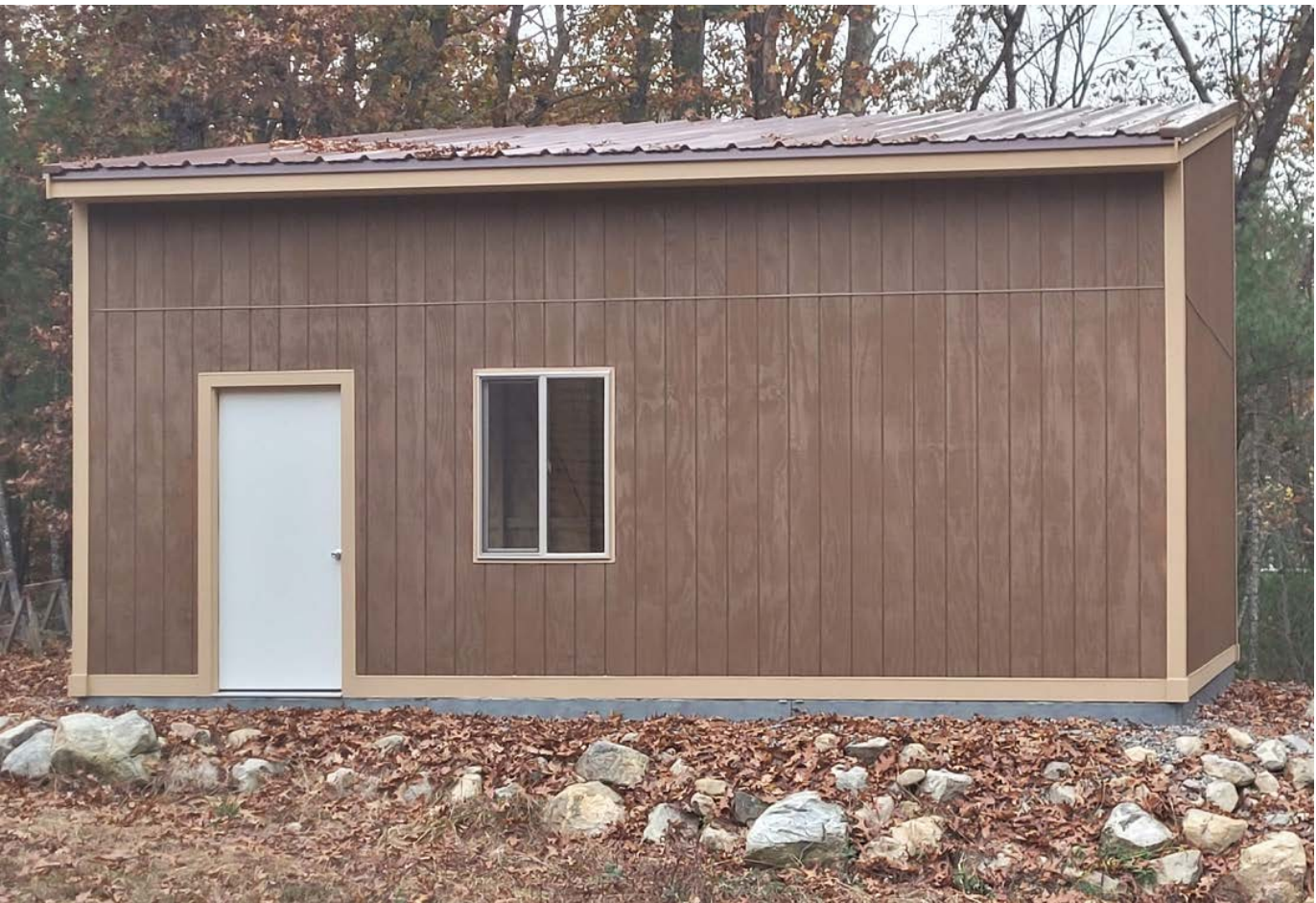
20 Rowley Rd Boxford, New Barn – Side View (west)
