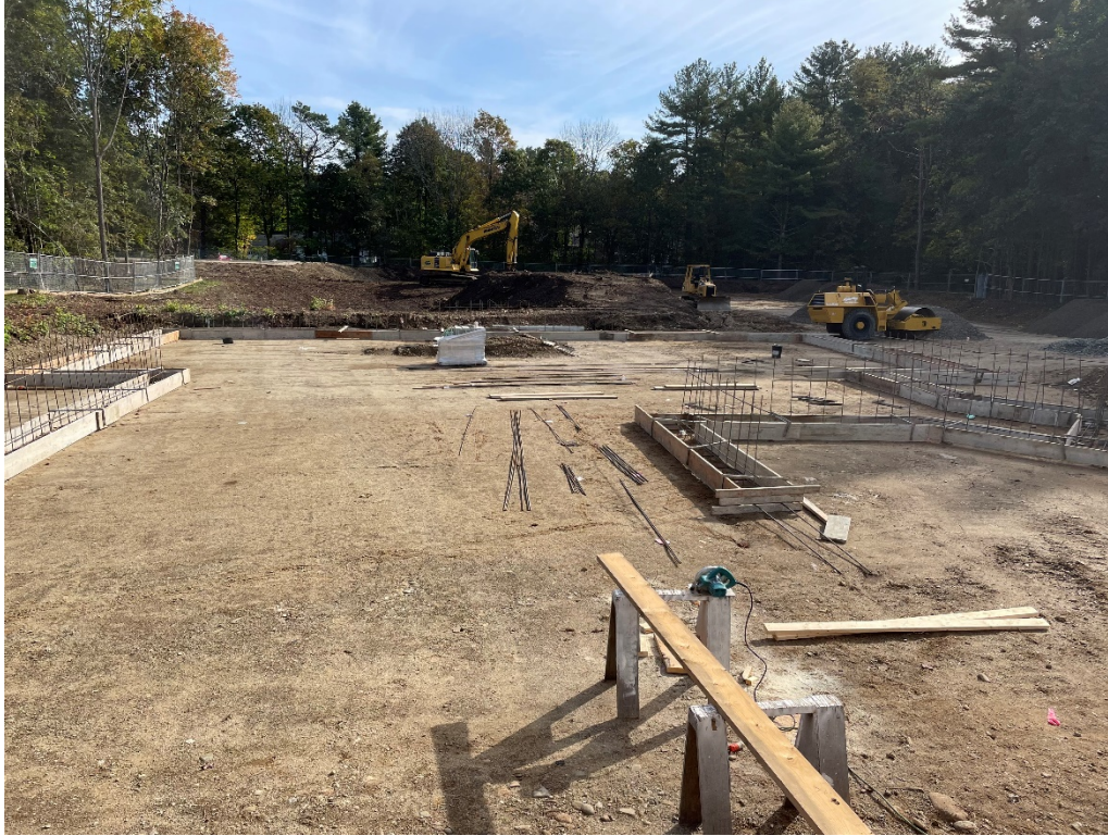
Figure 1 Forms for foundation footings.
