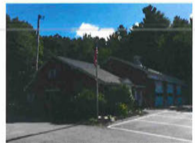
WEST FIRE STATION BUILDING EXTERIOR
