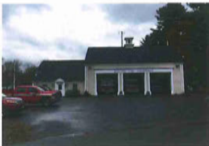
EAST FIRE STATION - 6 MIDDETON RD
