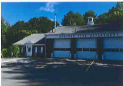
WEST FIRE STATION - 585 MAIN ST
