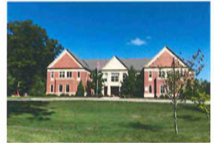
TOWN HALL - 7A SPOFFORD RD
