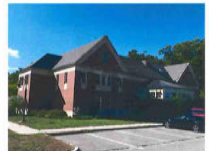
TOWN HALL - 7A SPOFFORD RD
