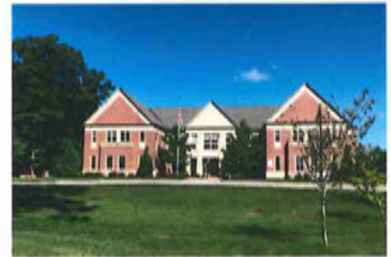
TOWN HALL - 7A SPOFFORD RD
