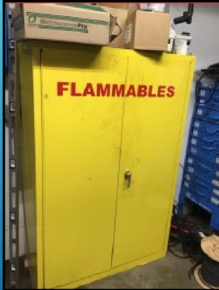
Inadequate Space for HazMat and Flammables
