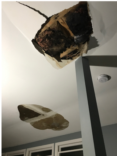
Tree damage to roof resulting in leak
