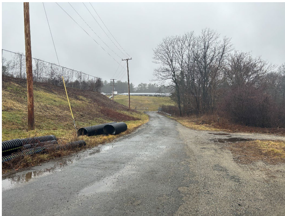
Figure 2 – DPW Access Driveway overview of driveway conditions. Photo taken facing northwest.
