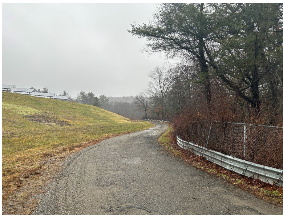
Figure 4 – DPW Access Driveway overview of driveway conditions along curved corridor. Photo taken facing north.
