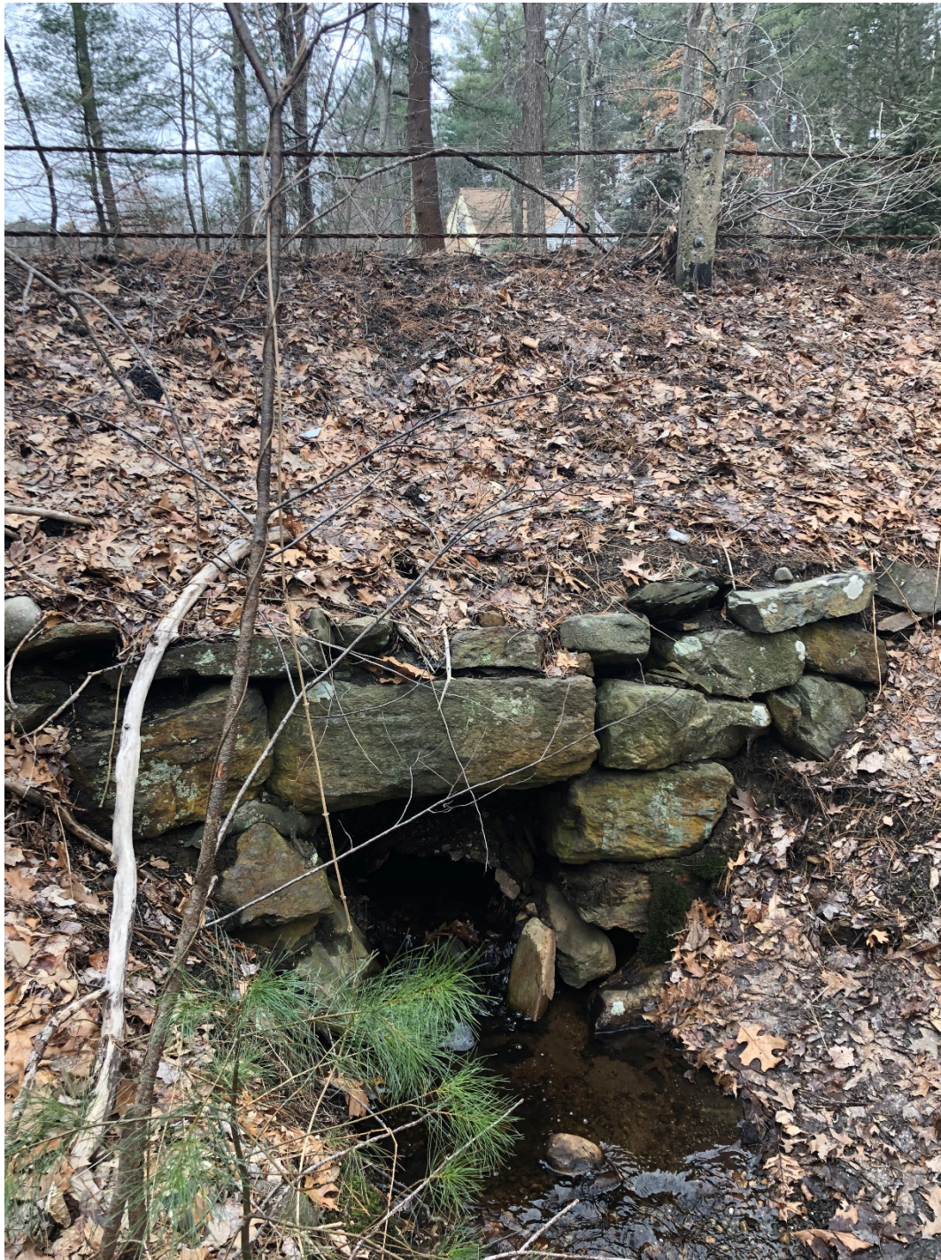
Figure 2: Culvert pipe end and stone reinforcement at downstream
