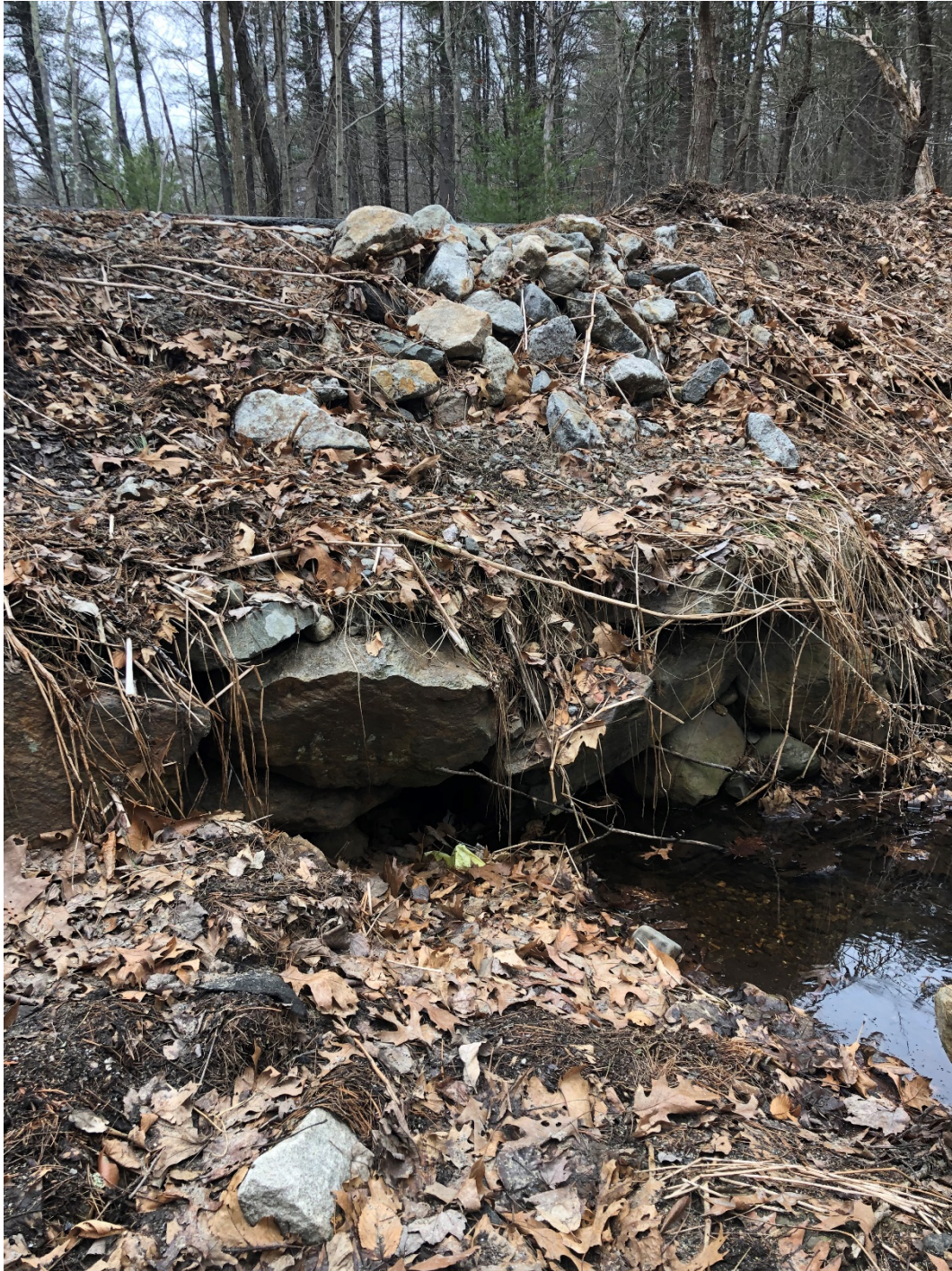
Figure 4: Upstream culvert end, located on the south side of Willow Rd.
