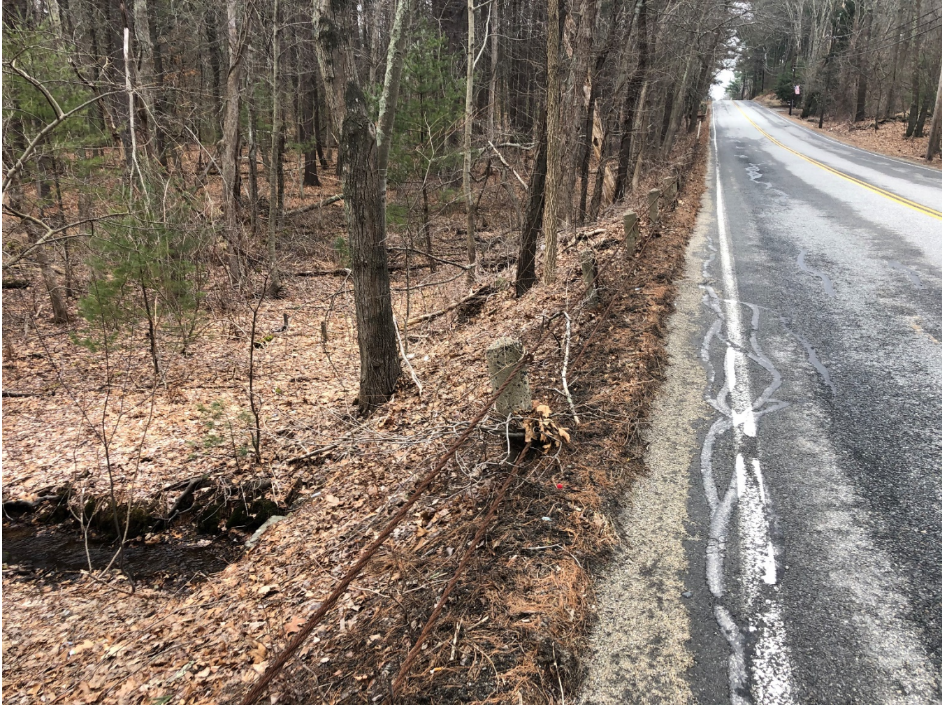
Figure 1: Culvert outlet on the north side of Willow Rd, photo taken facing east
