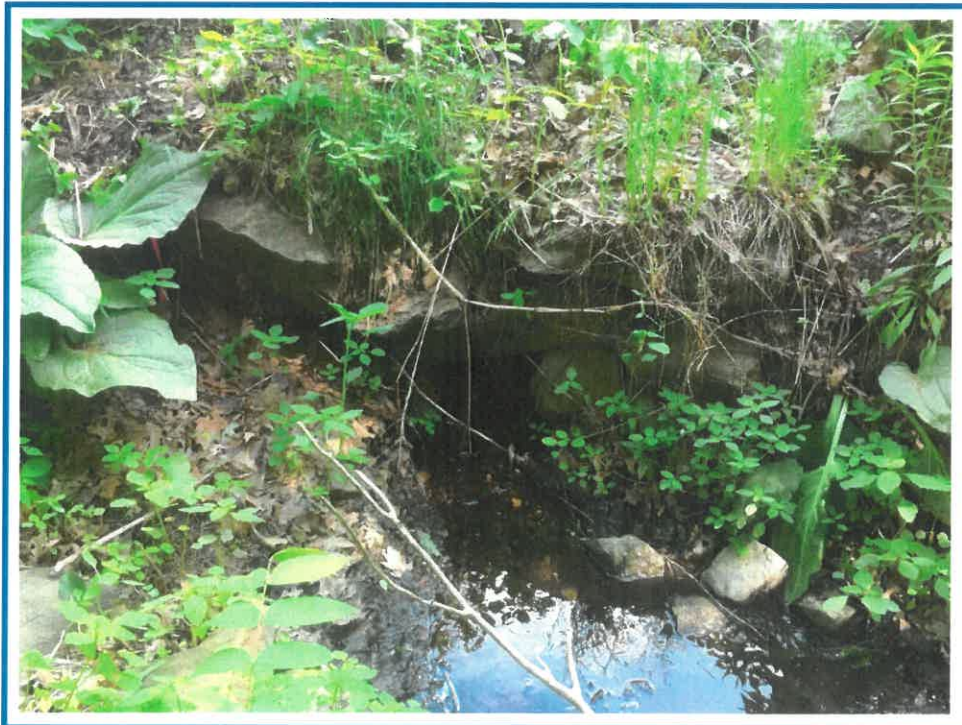
Upstream Culvert Entrance
