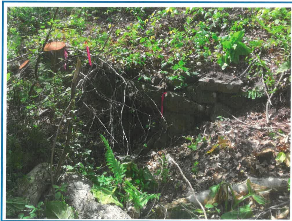
Downstream Culvert Exit
