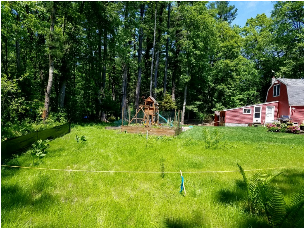
Photo #2: Structures partially within 25' NDZ – 30 May 2018
