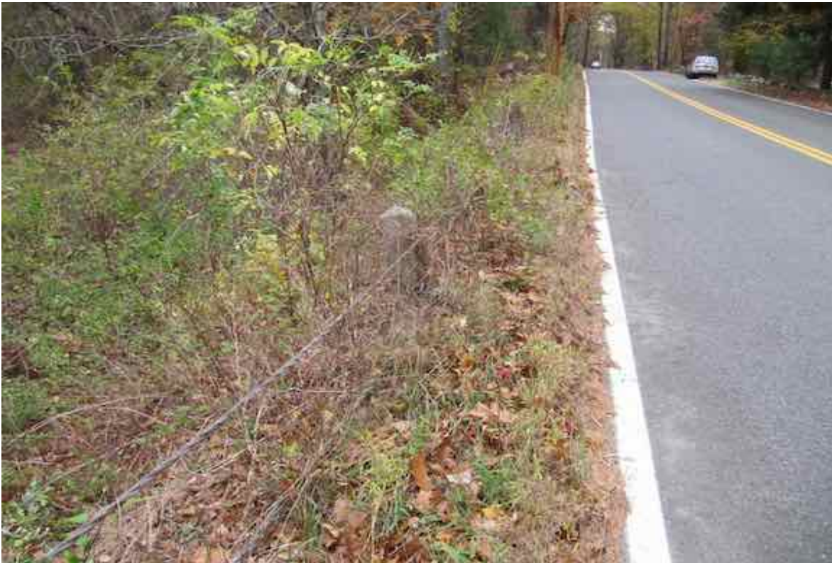
Photo E. Northerly view of guardrail adjacent to wetland E. Photo by B. Prokop 11/5/17.
