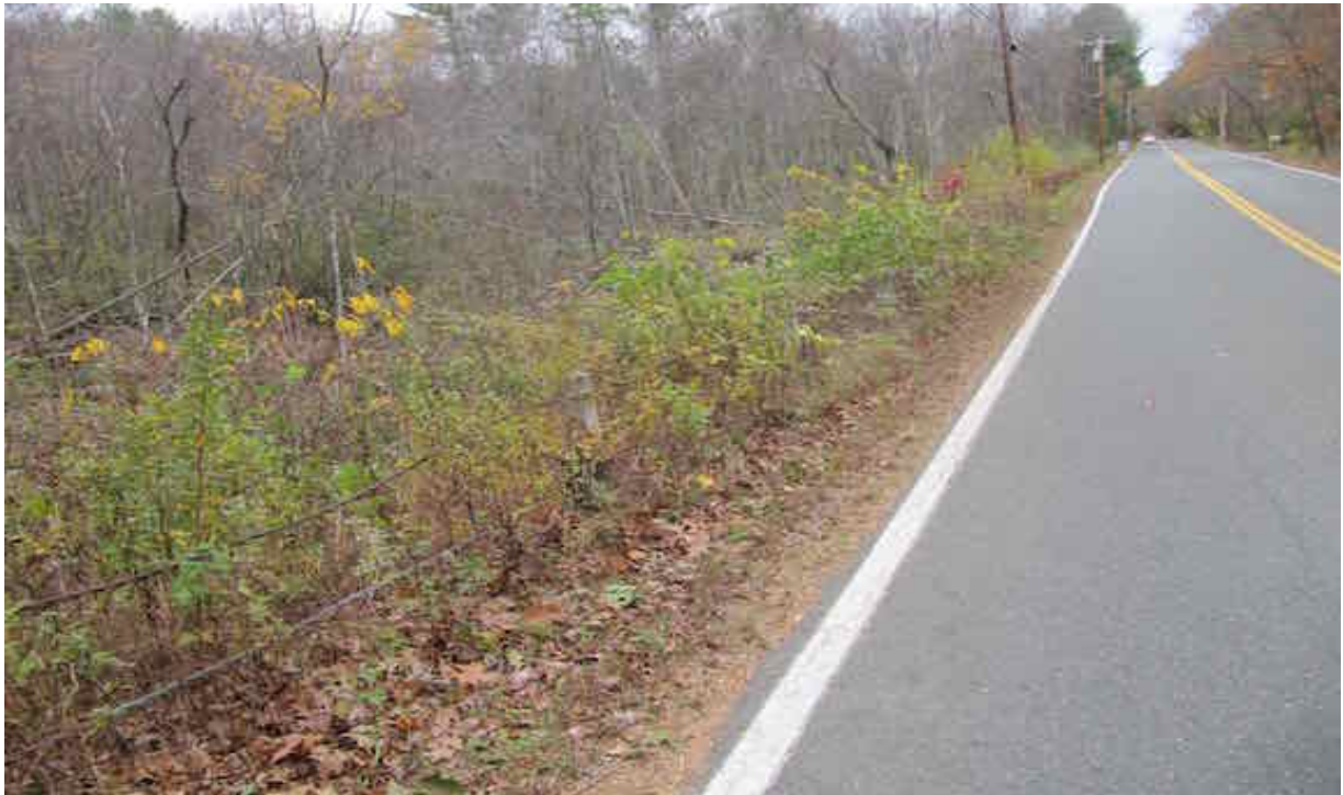
Photo J. Southerly view of guardrail adjacent to Wetland J. Photo by B. Prokop 11/5/17.
