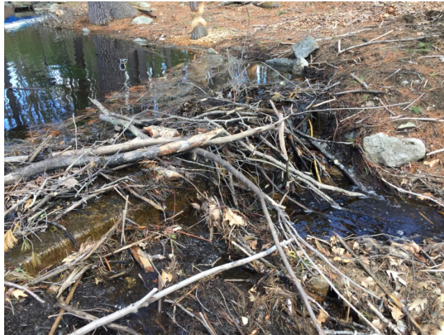
Close-up of dam and spillway with debris 4-20-18.
