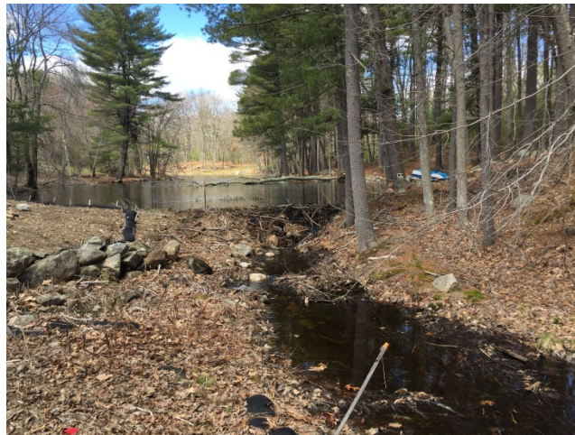
View looking upstream of spillway and dam, 4-20-18.
