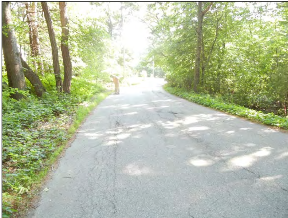
Photo No. 2 – Valley Road looking northeast
