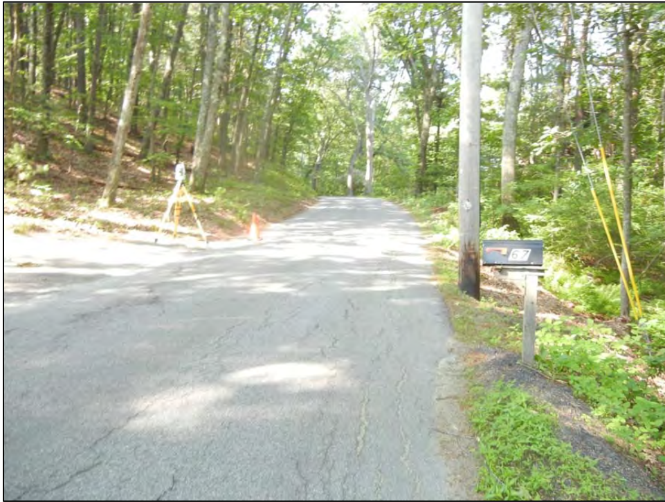
Photo No. 1 – Valley Road looking southwest
