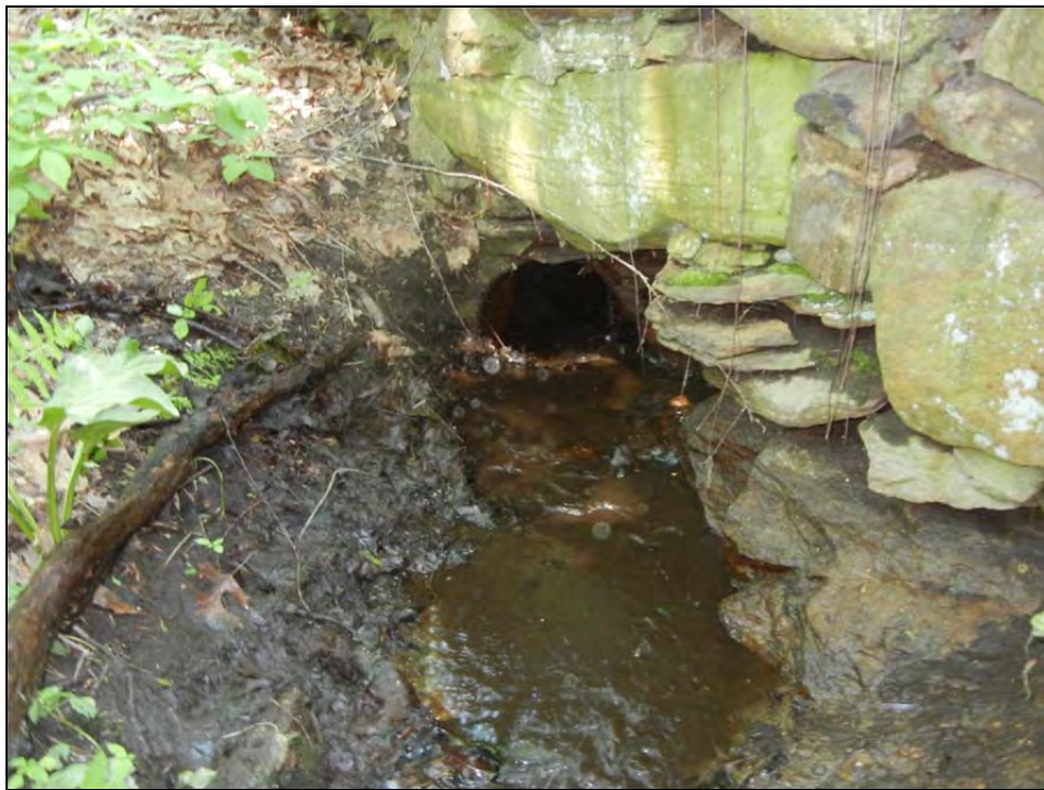
Photo No. 6 – 18-inch corrugated metal pipe upstream invert
