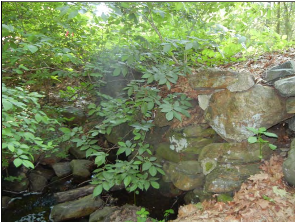
Photo No. 10 – West (downstream) headwall
