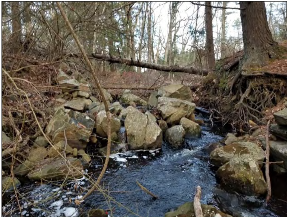
Photo No. 8 – Upstream mill race dike/bank of main Fish Brook channel
