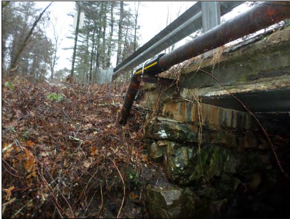
Photo No. 9 – Southwest bridge quadrant – 4 inch steel gas main
