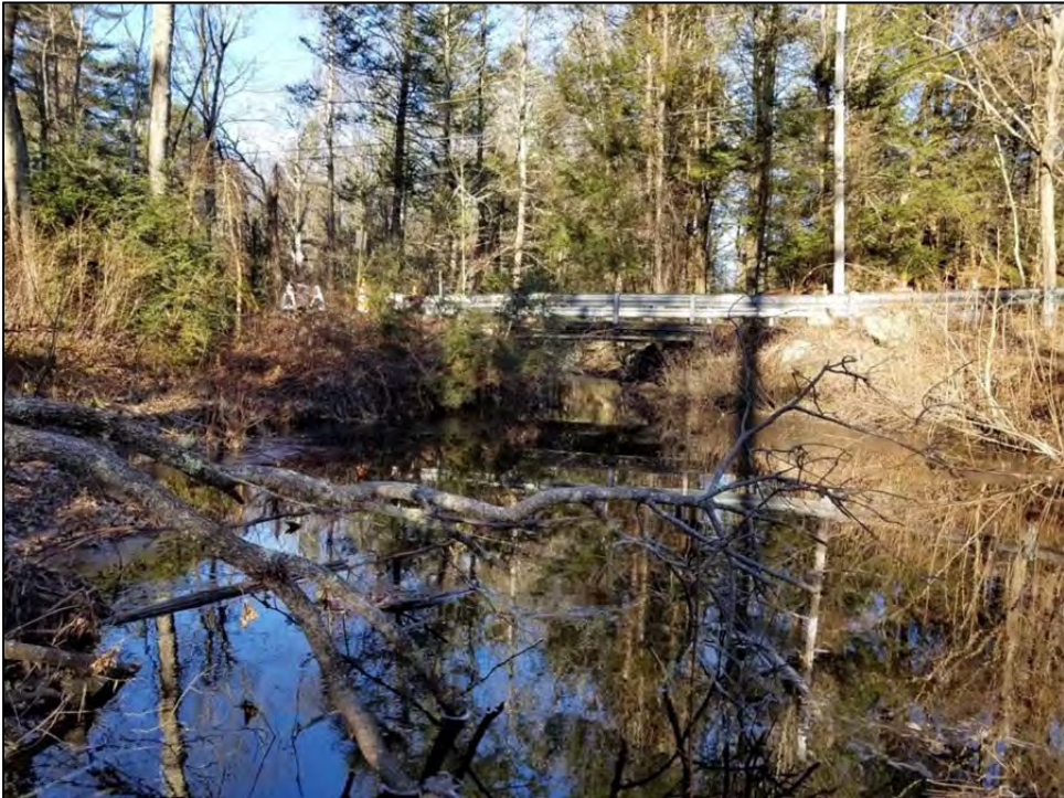
Photo No. 6 – South elevation
