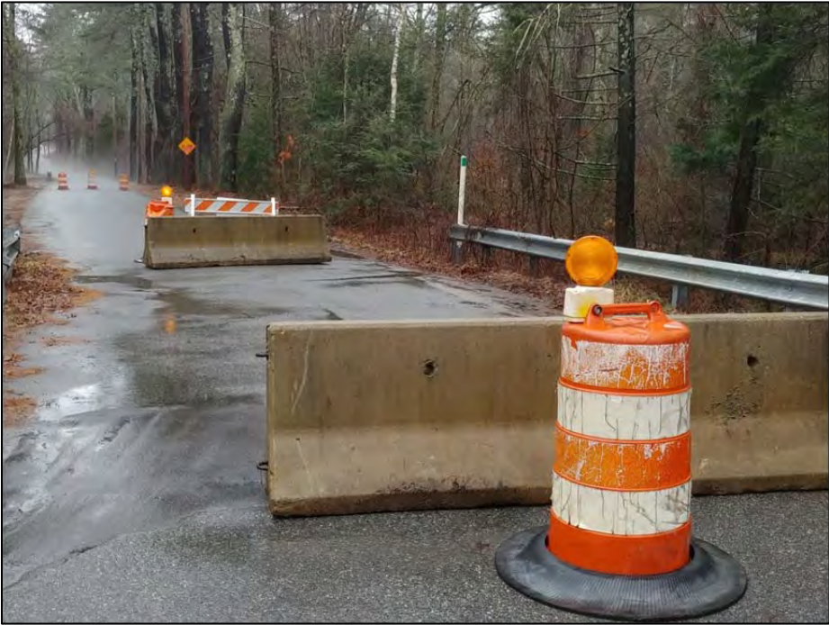
Photo No. 2 – Lockwood Lane looking west
