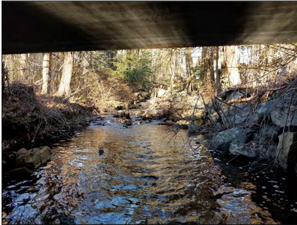
Photo No. 3 – Looking north at upstream channel
