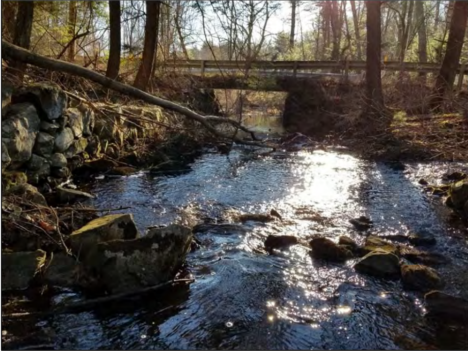
Photo No. 5 – North elevation
