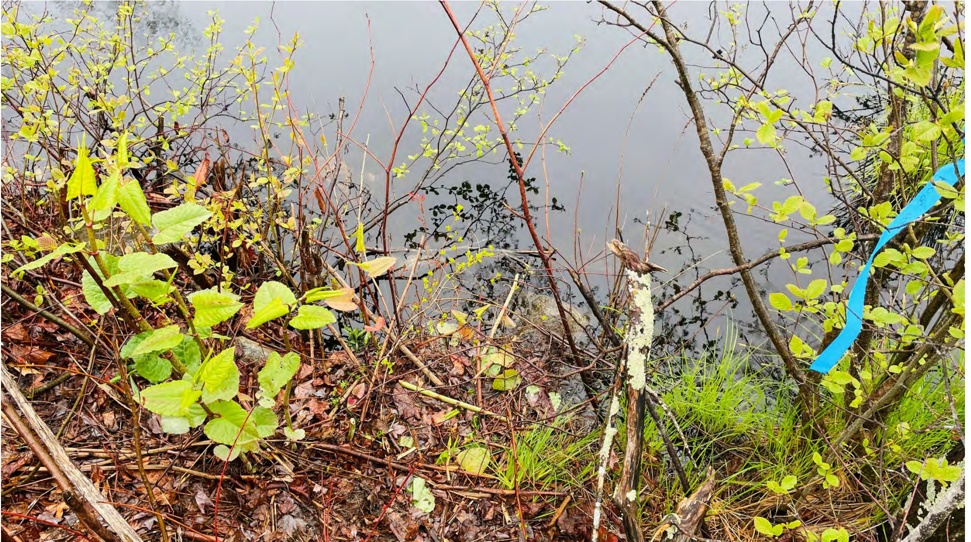
Photo 3 – Close up view of bottom of rip rap slope to be temporarily altered. Bank Flag TOB 8 is visible to the right.
