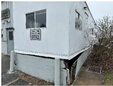
Existing DPW Structure
