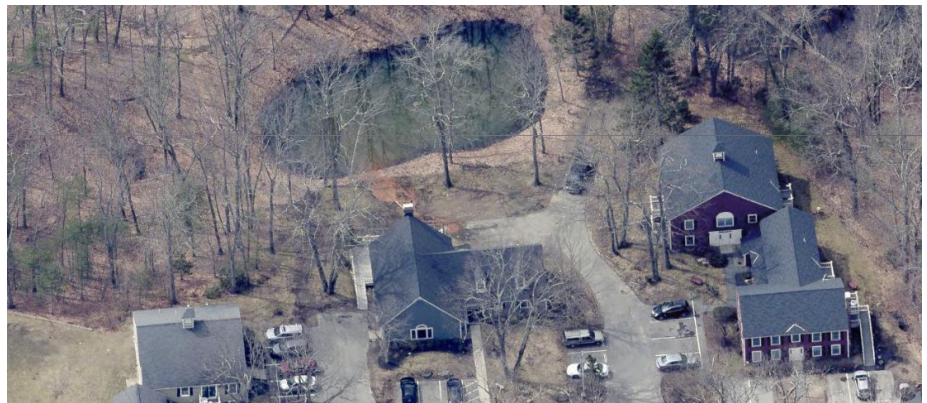
Aerial view of the existing Fire Pond at 50 Four Mile Village, Boxford
