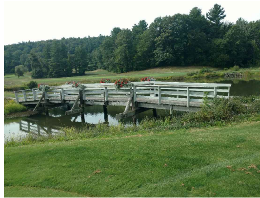
A SITE PHOTO SCALE: NTS
