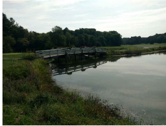
A SITE PHOTO SCALE: NTS
