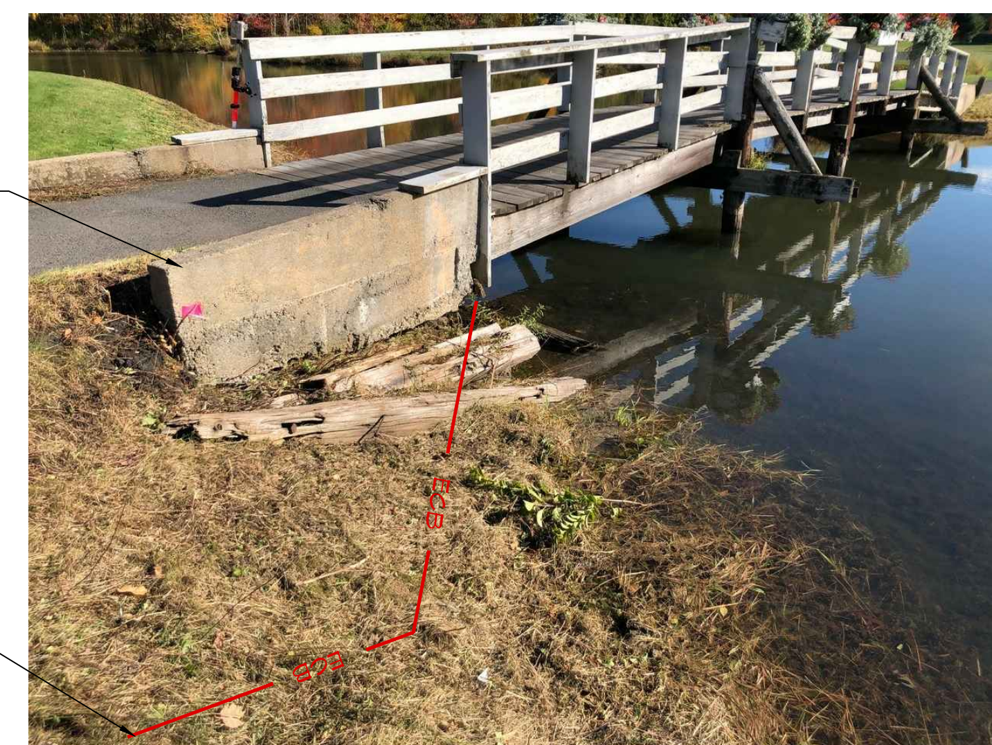
EXISTING CART PATH BRIDGE - PHOTOGRAPH #1
