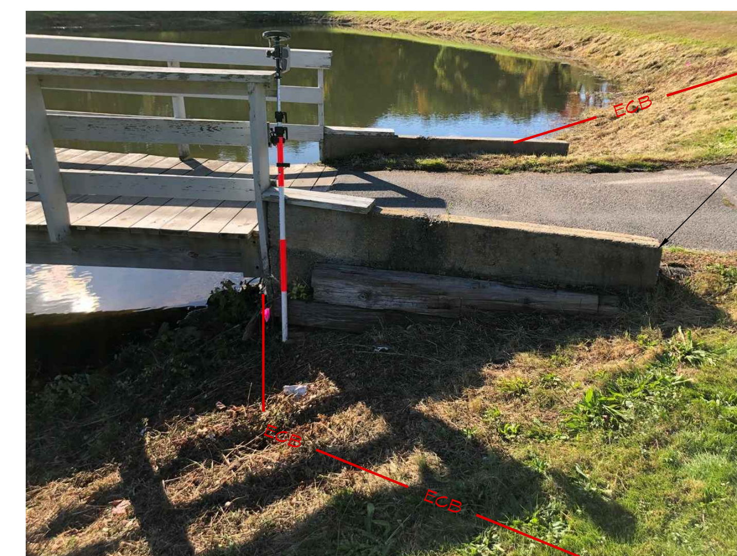
EXISTING CART PATH BRIDGE - PHOTOGRAPH #1
