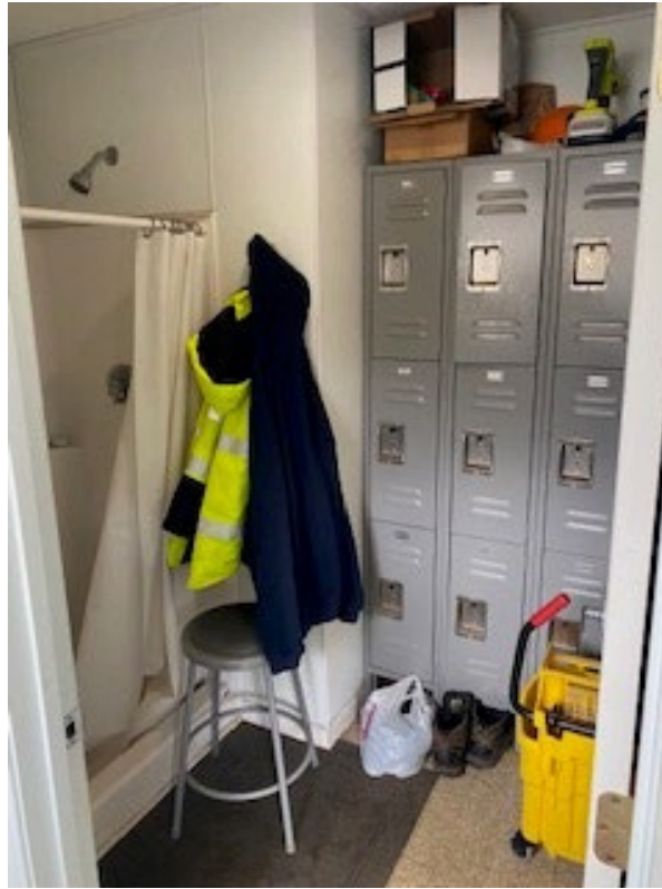
Shower and Locker Room Doubles as a Janitor's Closet
