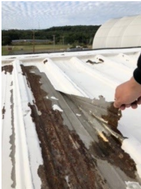
Rusted metal frame and roof exposes building to rain, snow and ice
