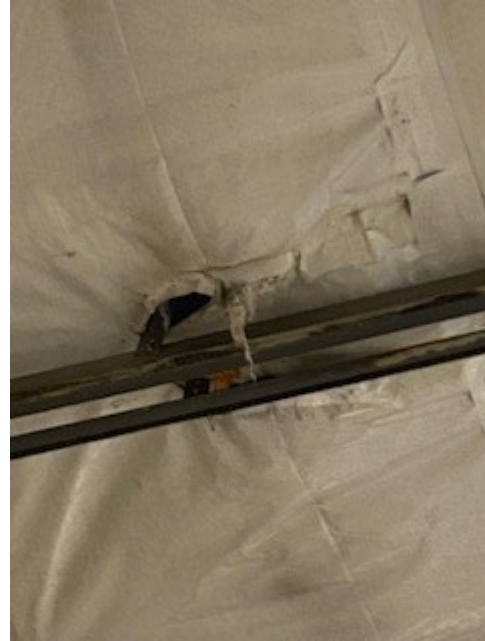
Leaking Water Causes excessive moisture, mold and damage
