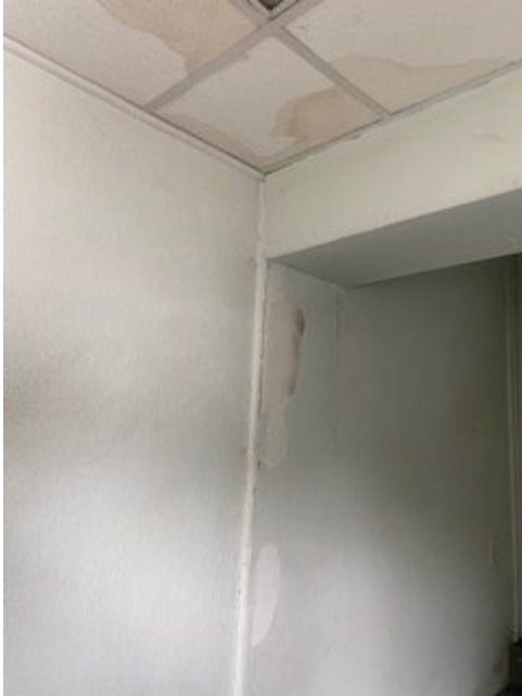
Leaking Water Causes excessive moisture, mold and damage
