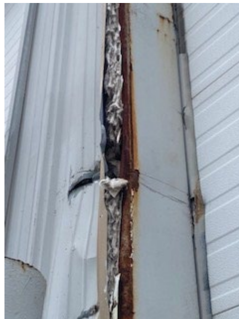
Rusted metal frame and roof exposes building to rain, snow and ice
