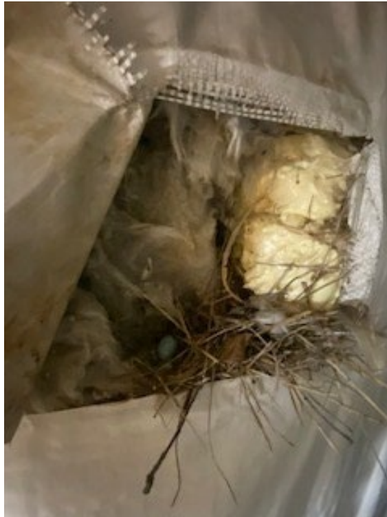
Holes in the walls allow for animals to nest throughout the building
