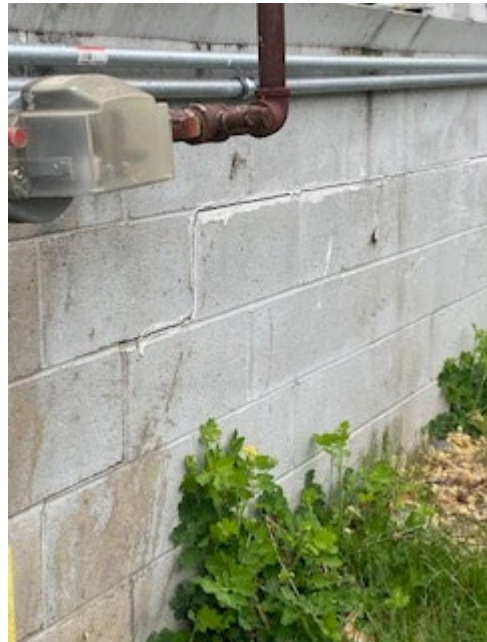
Cracks in the foundation and slab due to poor subsoil cause increased risk of instability of building
