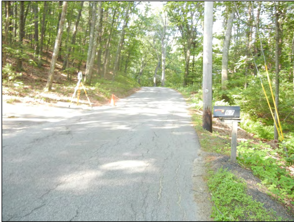
Photo No. 1 – Valley Road looking southwest
