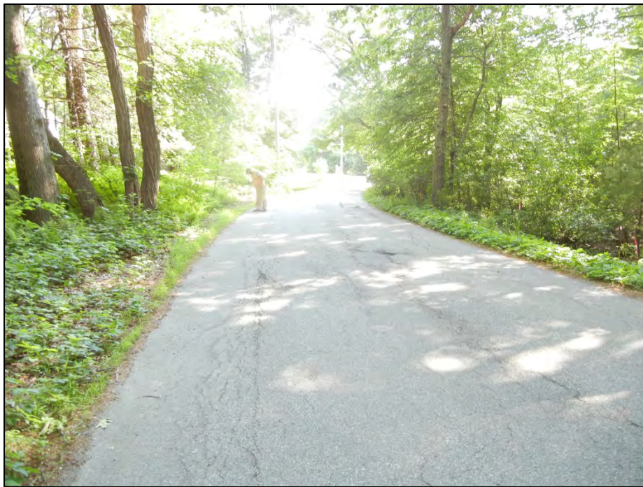
Photo No. 2 – Valley Road looking northeast
