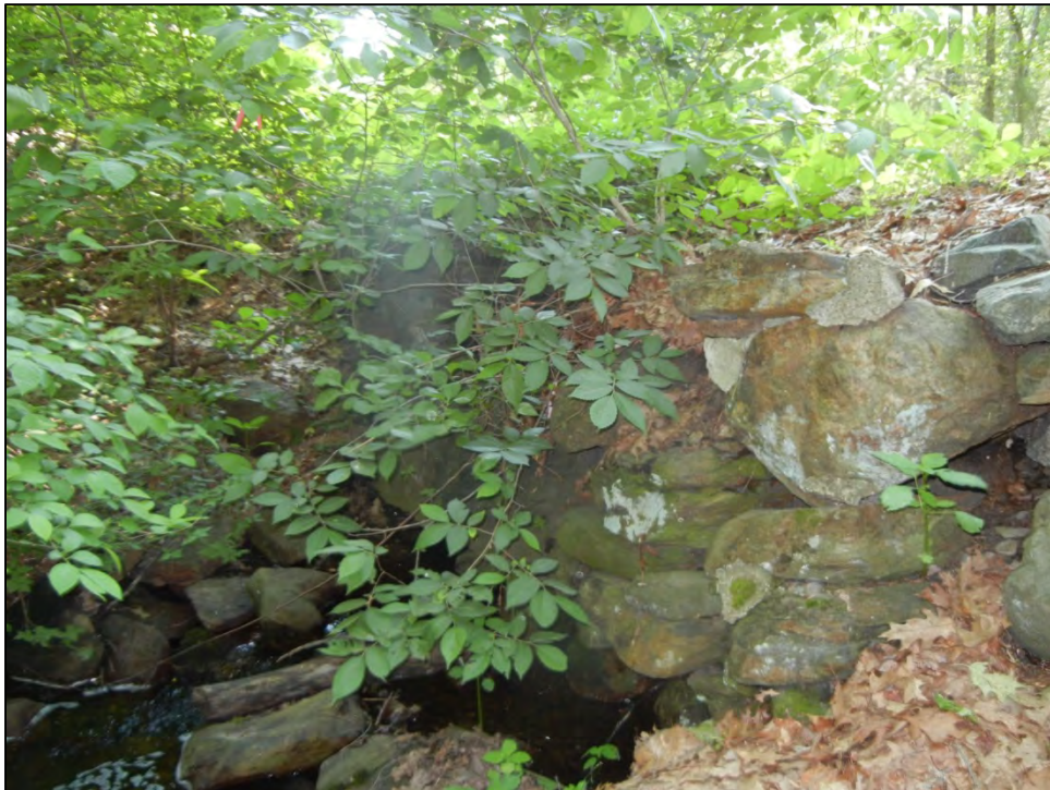
Photo No. 10 – West (downstream) headwall
