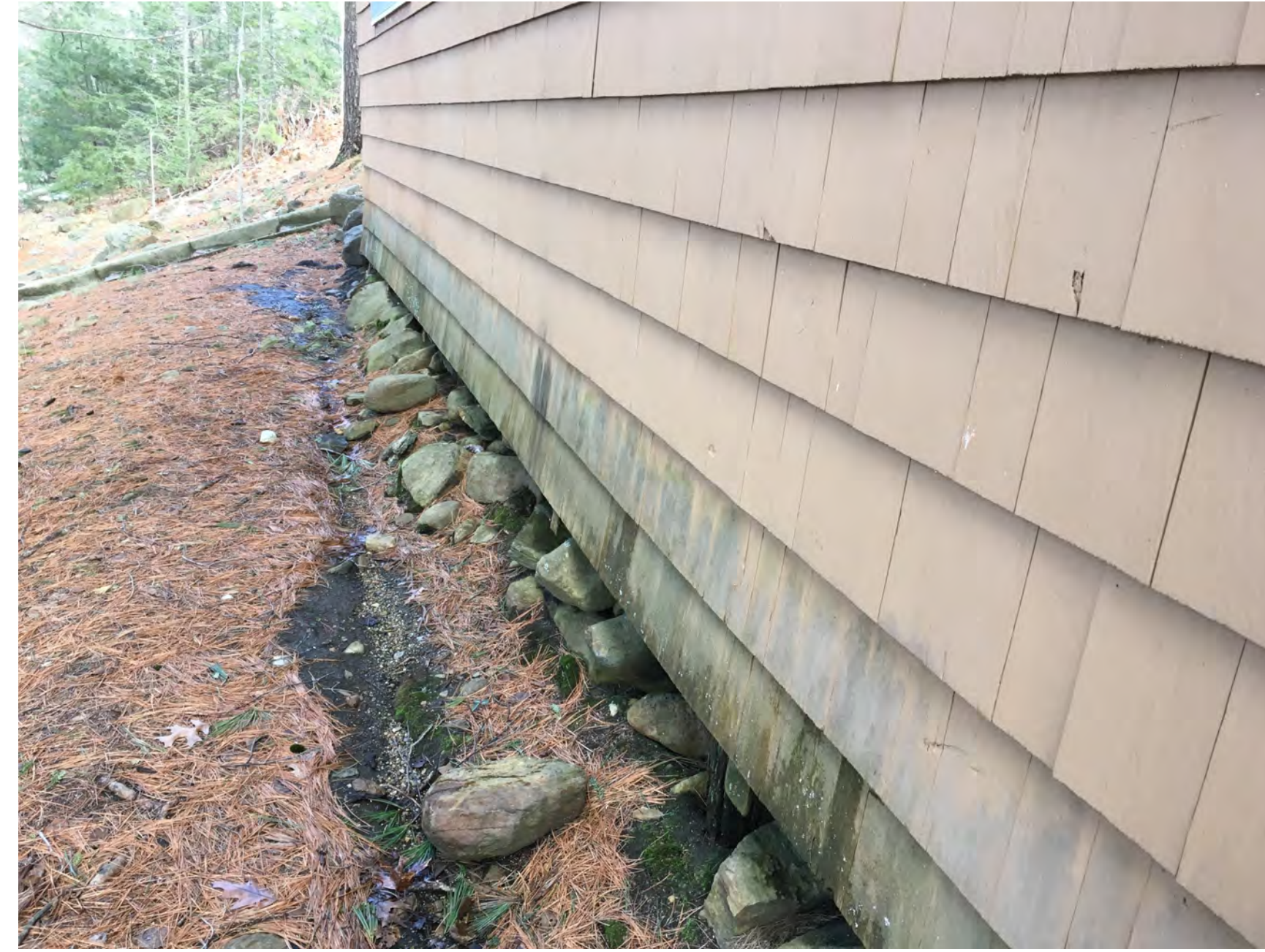
View along back of dining hall which will be removed
