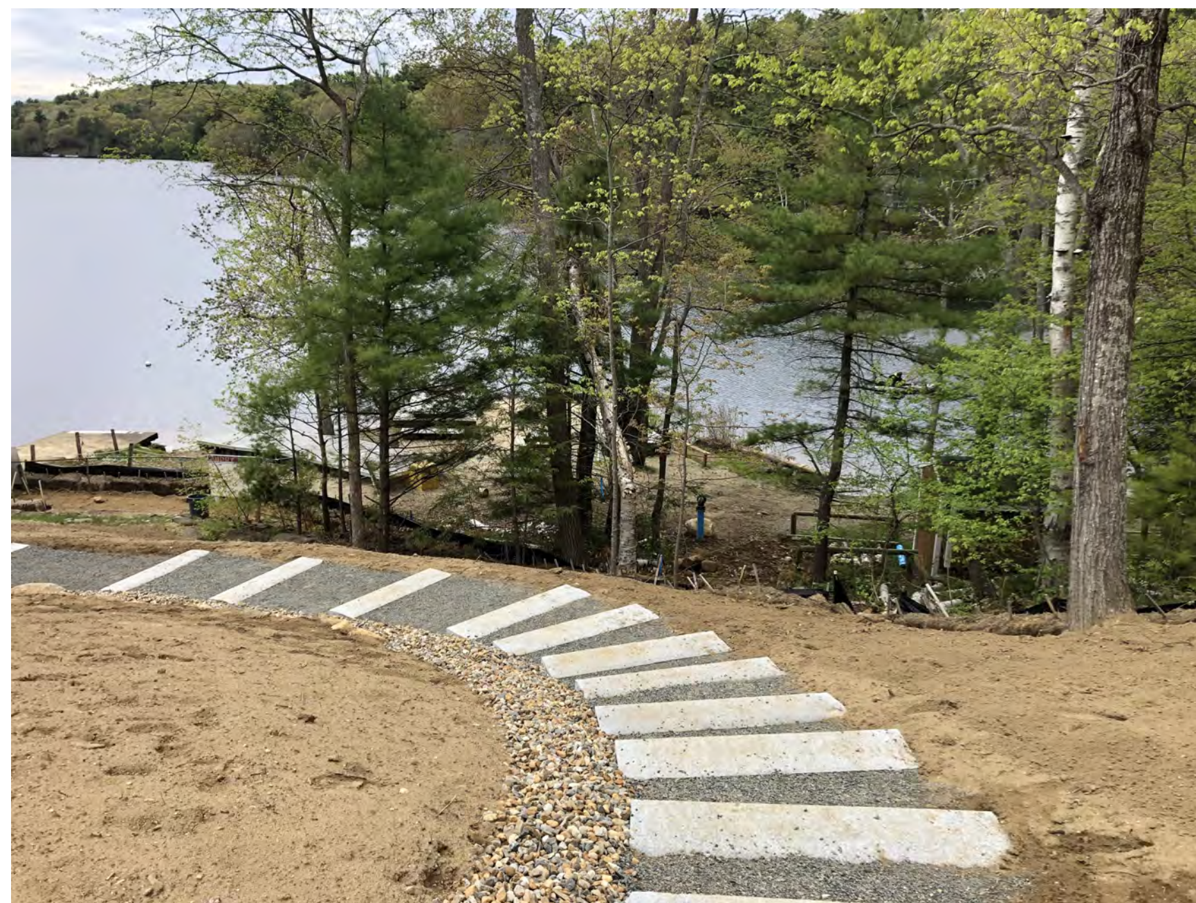
Hydrant on pipe visible at bottom of slope
