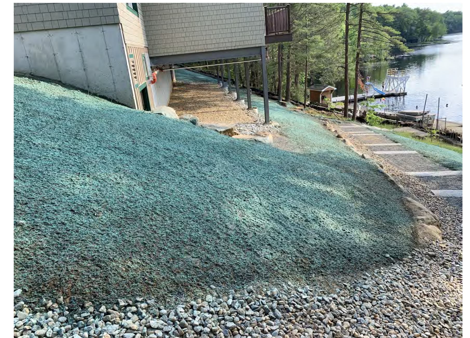
Area where trees were removed hydroseeded with native slope mix
