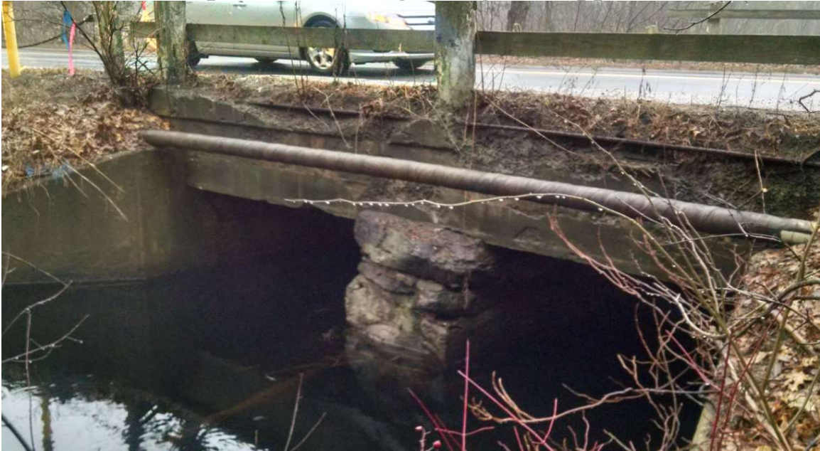
Photo 1: General elevation (looking southwest).
