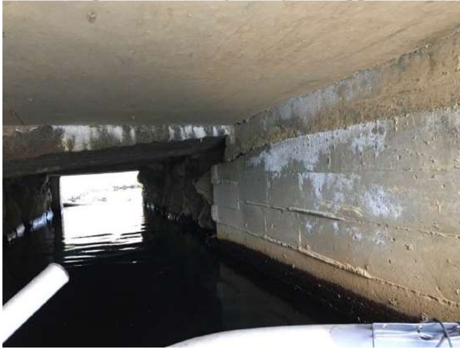
Photo 3: Underside of bridge, looking west
