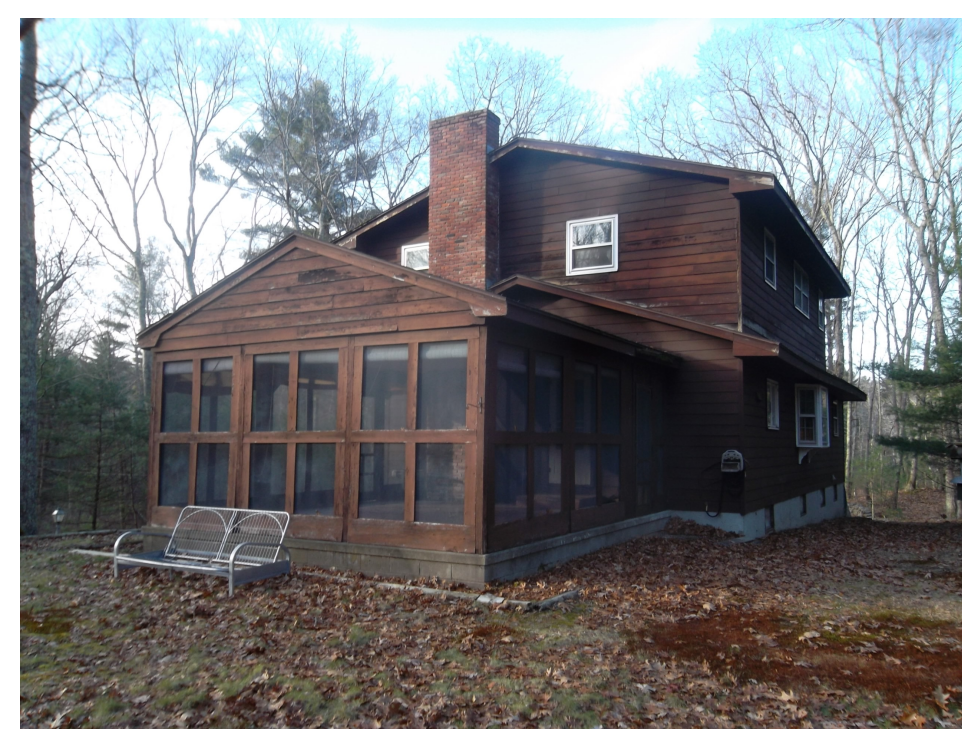
EXISTING CONDITIONS PHOTO
