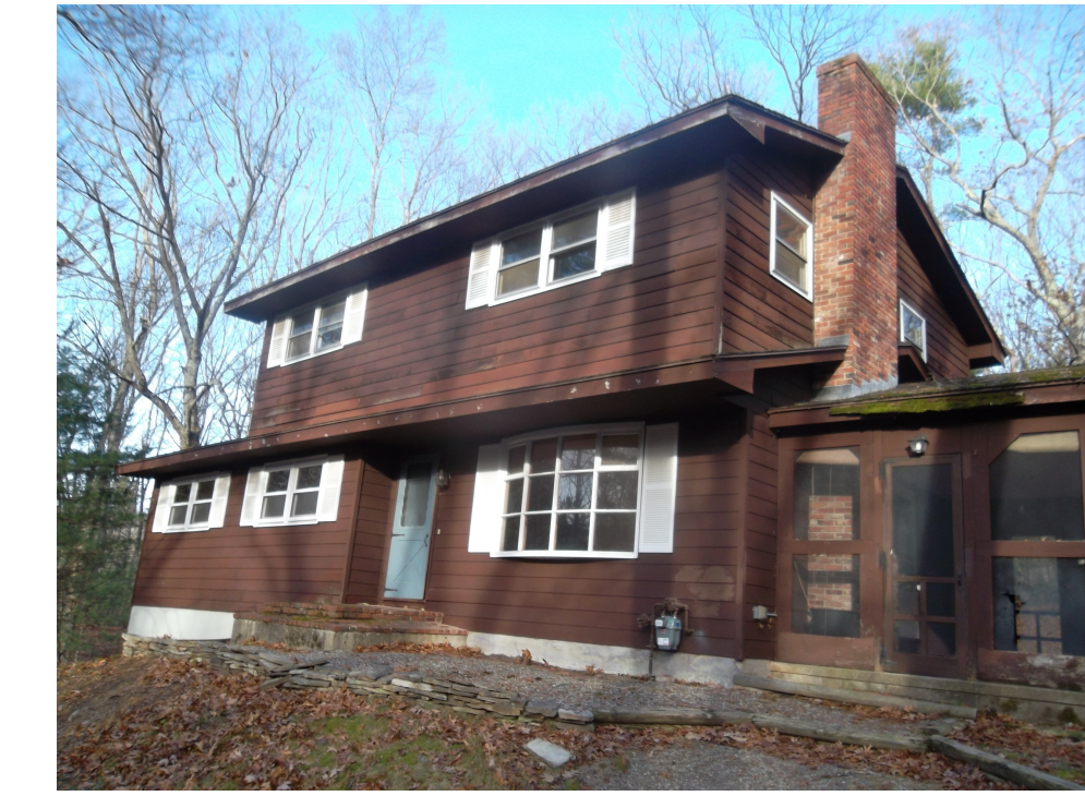
EXISTING CONDITIONS PHOTO
