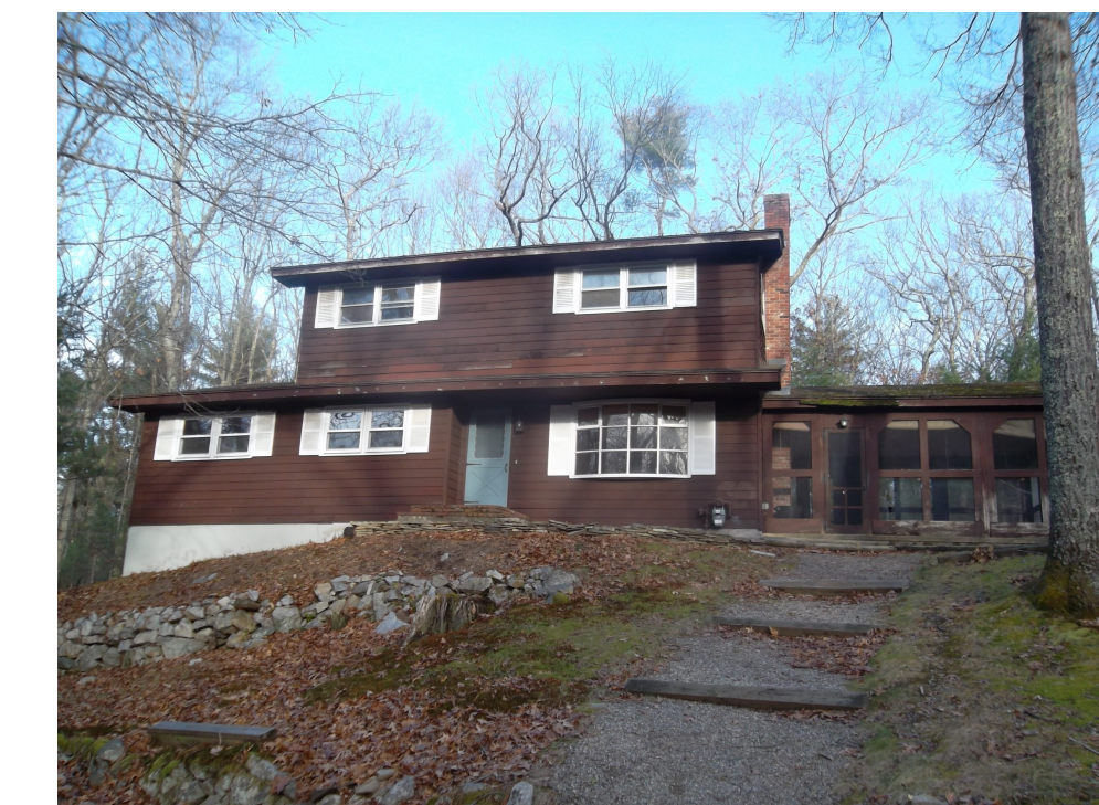
EXISTING CONDITIONS PHOTO
