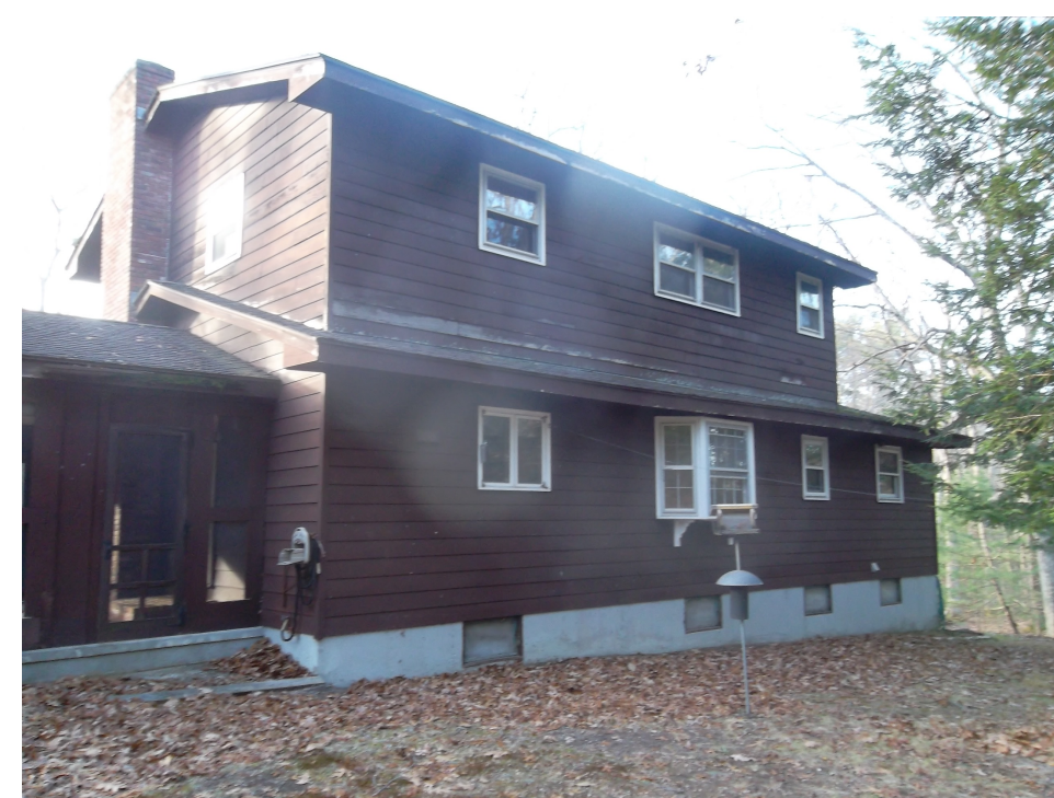
EXISTING CONDITIONS PHOTO
