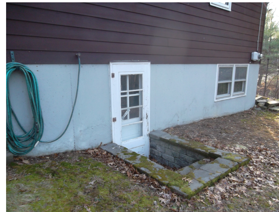
EXISTING CONDITIONS PHOTO
