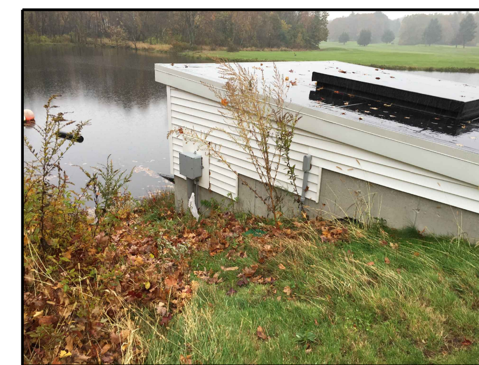
PHOTOGRAPH #4 PUMP HOUSE
