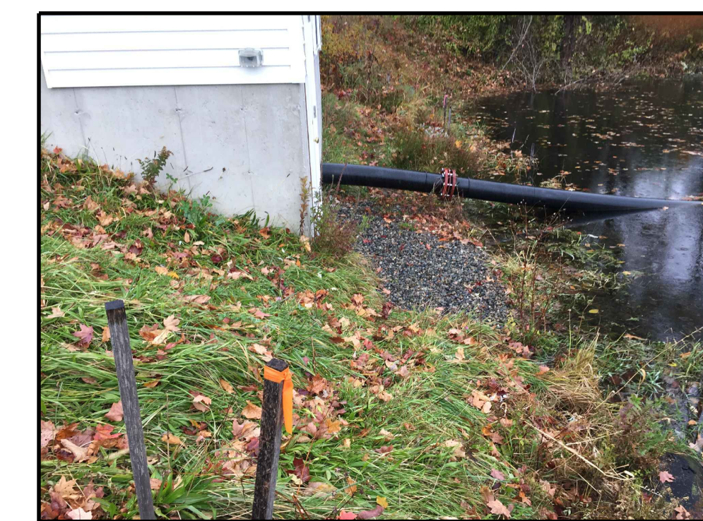
PHOTOGRAPH #5 PUMP HOUSE AND INTAKE PIPE
