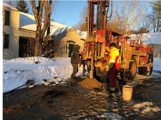
Typical Drill Rig Setup
