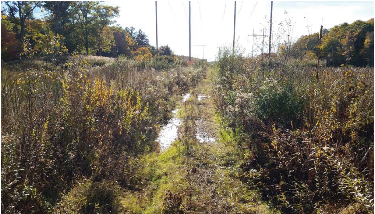
Photo 1: View of existing access road on the 394 Transmission Line ROW located off Baker Street. This access road will require temporary matting to access Structures 154 through 157. Facing southeast.
