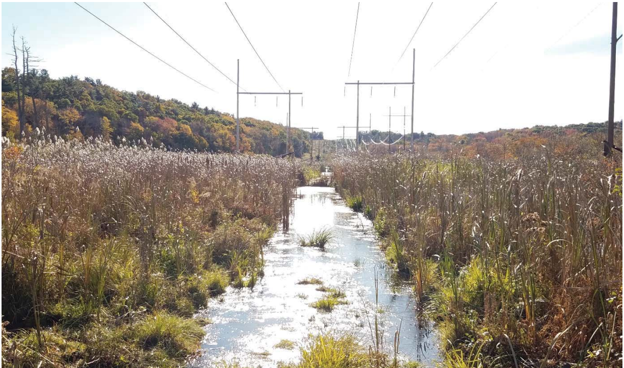
Photo 2: View of existing access along ROW. Best Management Practices will be used when crossing the wetland to access Structures 154 through 157. Facing southeast.
