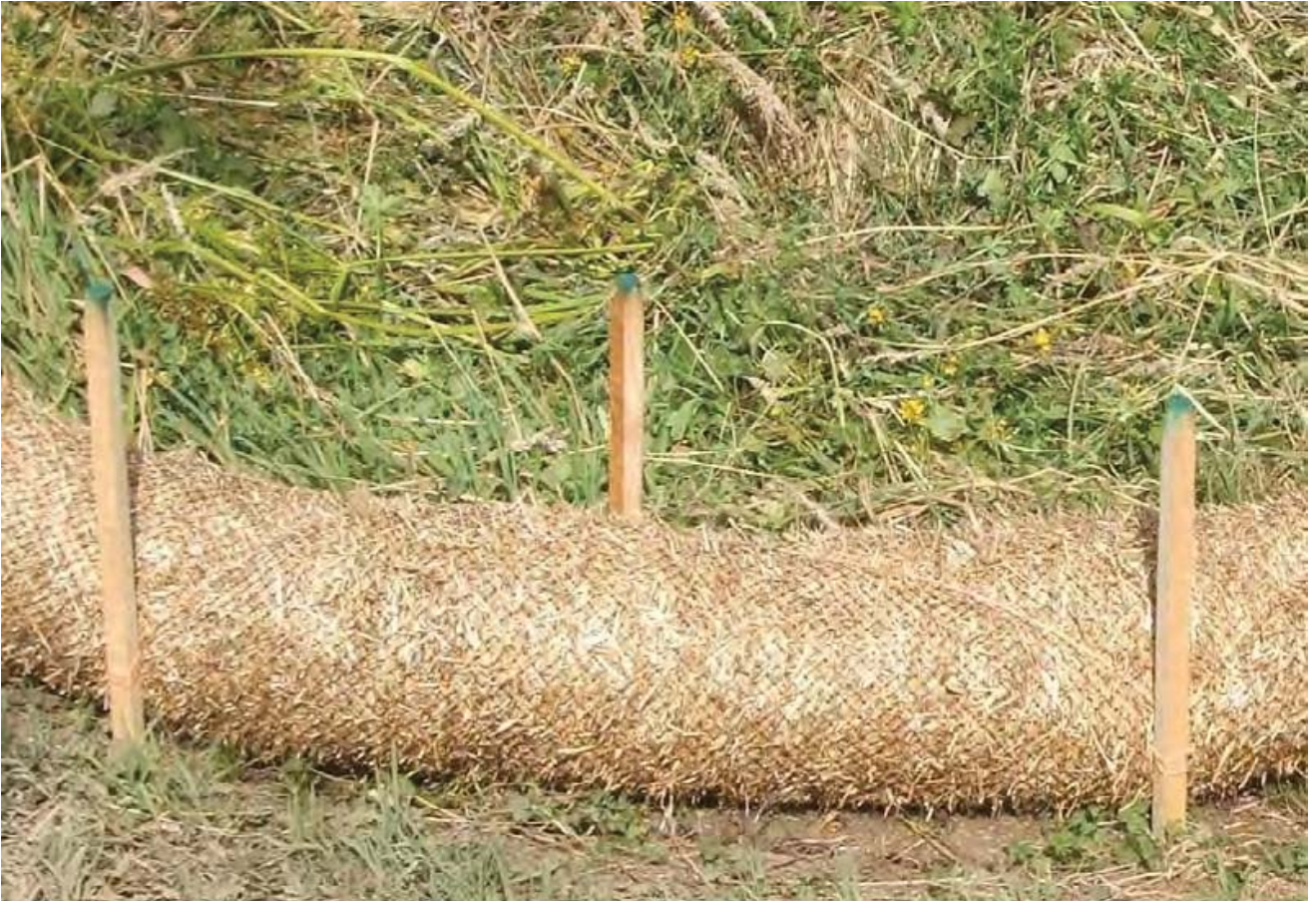
STRAW WATTLE – SHALLOW SLOPE ( \leq 4:1 ) (ALTERNATE STAKING)
