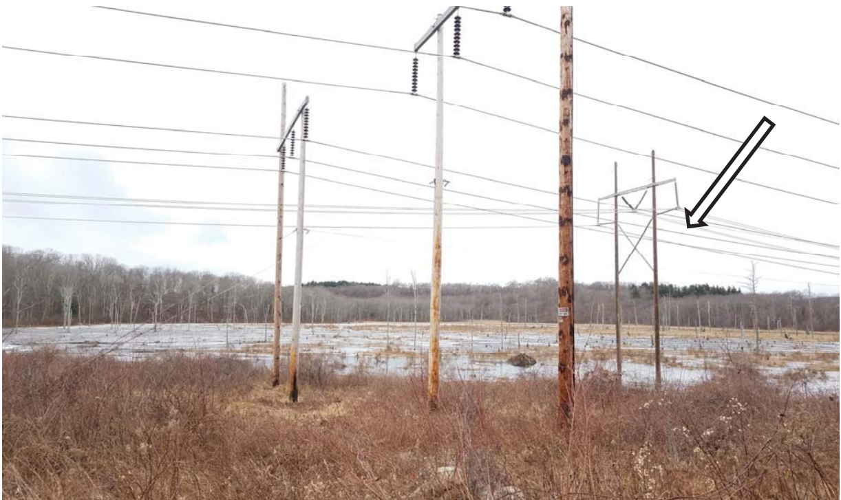
Photo 4: View of Structure 157 on the 394 Transmission Line. Facing northwest.
