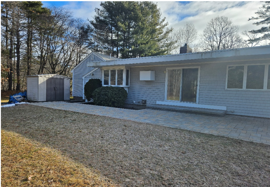
Photo #2: View of the back of the house with newly constructed patio. Photo taken by Hancock Associates Staff Scientist on February 7, 2024.
