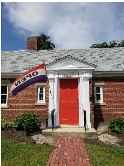
Newly painted door and trim
