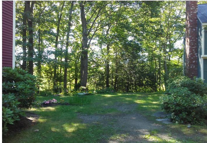
Photo # 3: Reverse angle from Photo #2. Drill rig access and area of piping connections.
