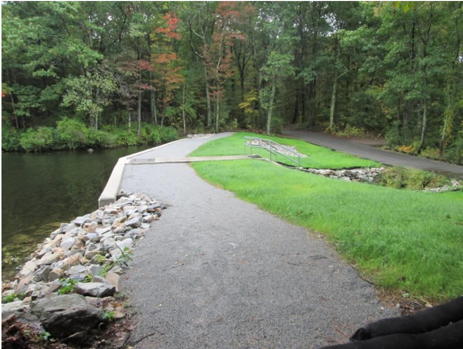
Figure 4. Stile Pond Dam.
