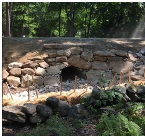
HIGHLAND ROAD DRAINAGE PIPE REPLACEMENT. CREDIT: TOWN OF BOXFORD
