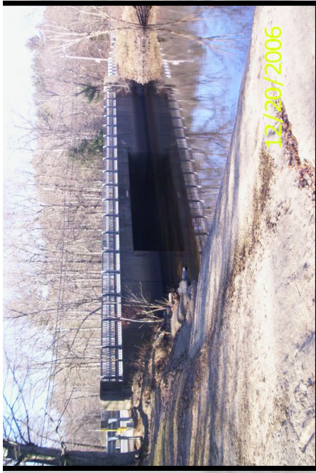
Typical water levels Gas distribution line suspended alongside the Towne Road Bridge over Fish Brook
