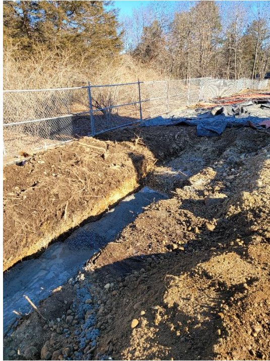
3. Electrical ductbank with concrete encasement
