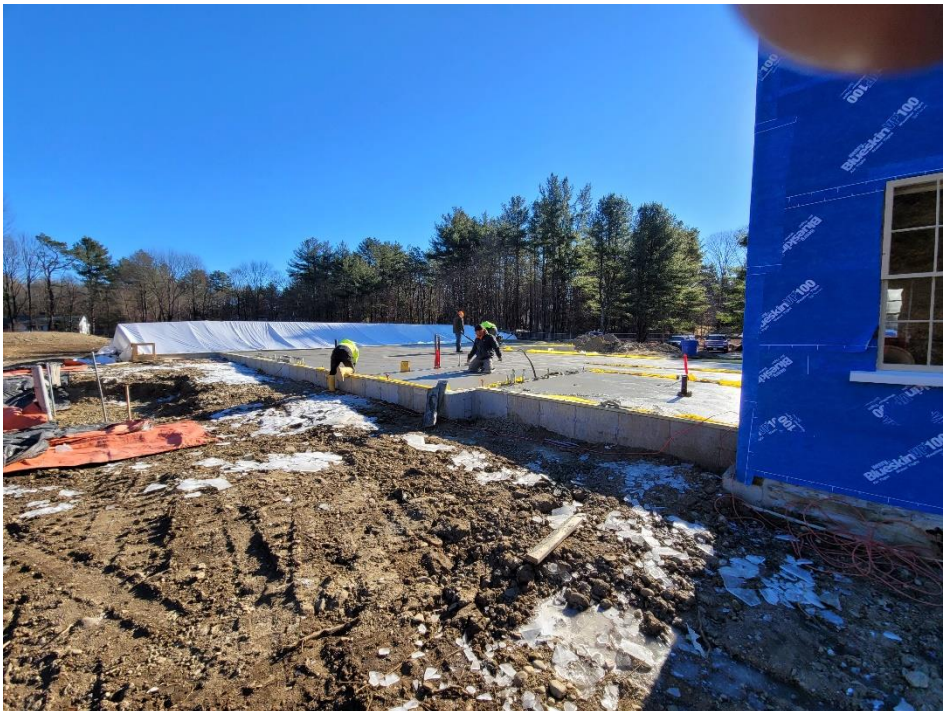
4. New concrete slab at Office wing, placed today, being finished in preparation for burning and tenting.
