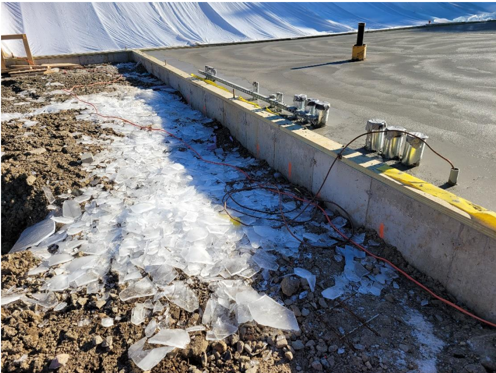
6. Stubs at Electrical Room and new slab in place
