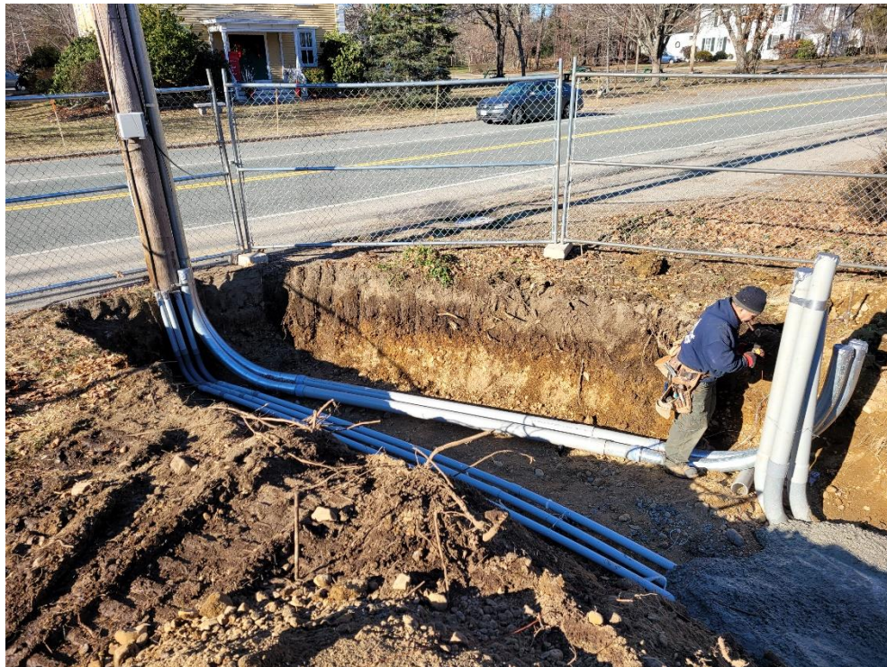
2. Electrical and Communication risers at base of existing pole; transformer risers in foreground
