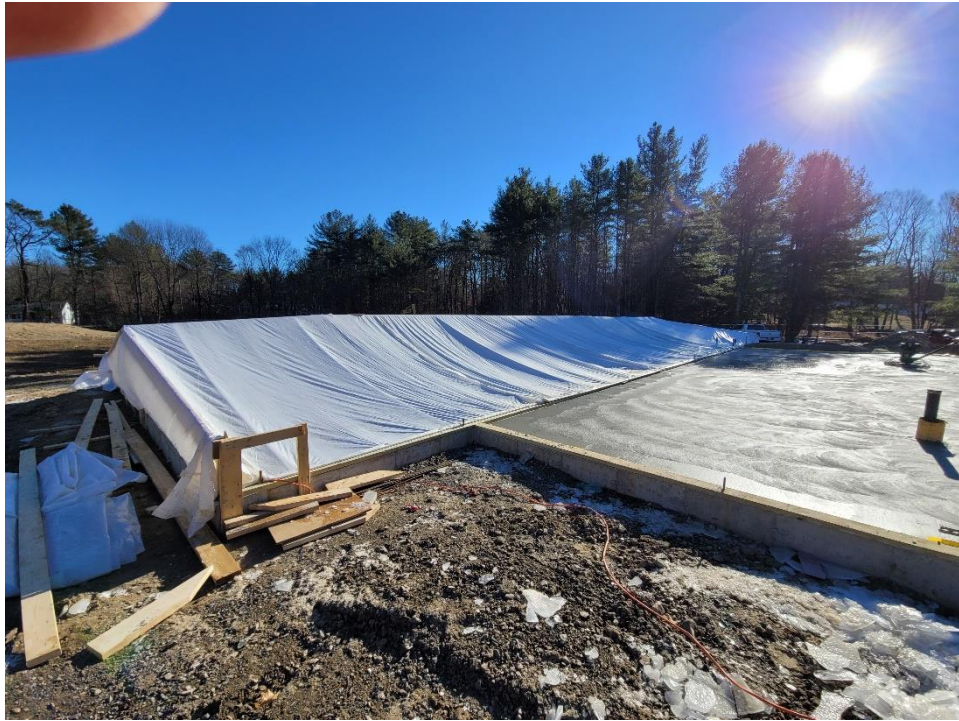
7. Tented Multipurpose/ Kitchen Wing slab; 7-day wet cure complete
