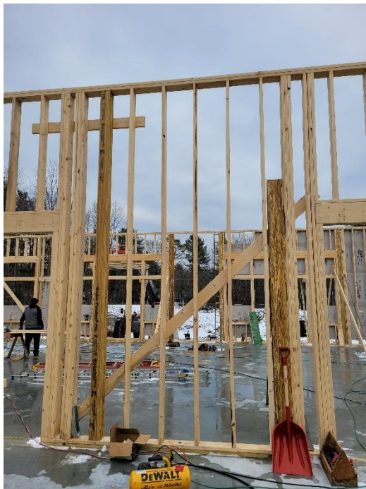
19. Parallam posts at interior wall to Multipurpose Room
