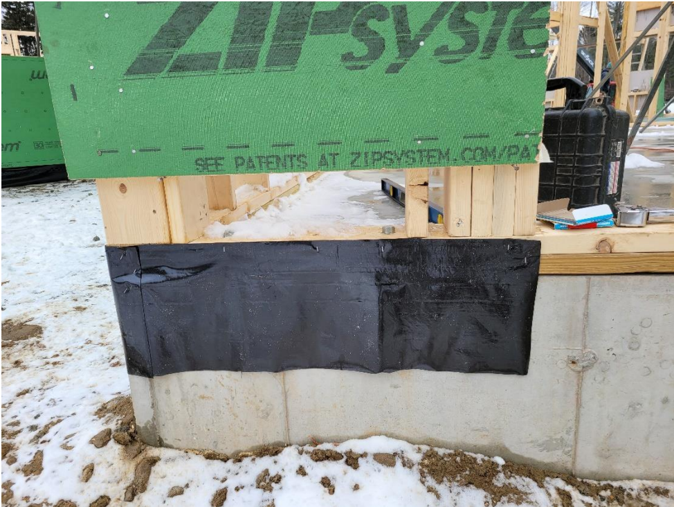
5. Detail of Ice & Water Shield at bottom plate- will wrap up face of P.T. blocking (not yet installed) per SKA-12b
