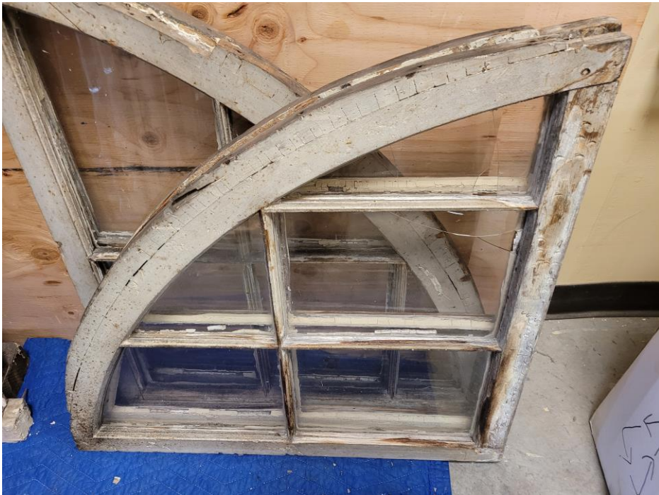
32. Attic window sash at restoration shop
