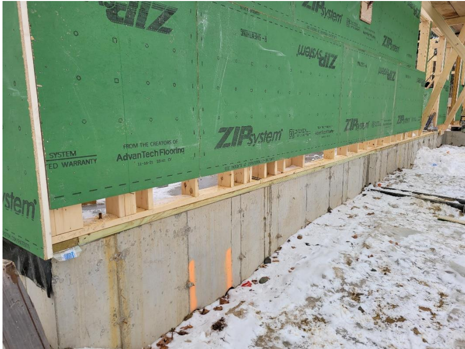
9. East Wall of Multipurpose Room with base detail per SKA-12b
