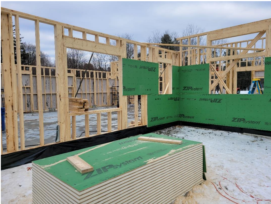
4. Installation of Zip R-Sheathing (R-6) with strip of Ice & Water Shield membrane at base per SKA-12a
