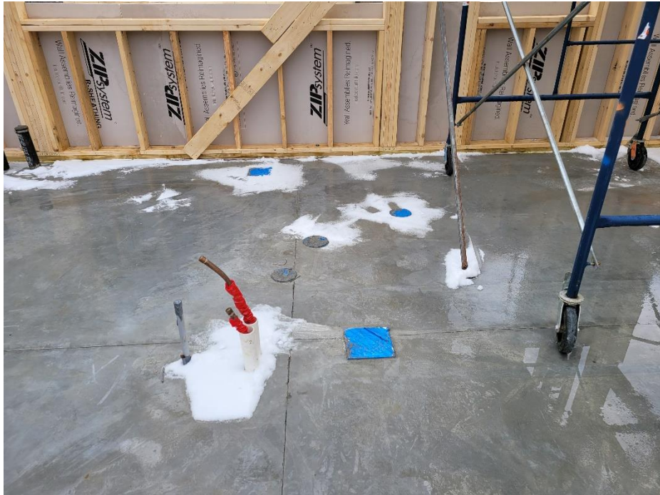
15. Floor drain (blue square) under island sink
