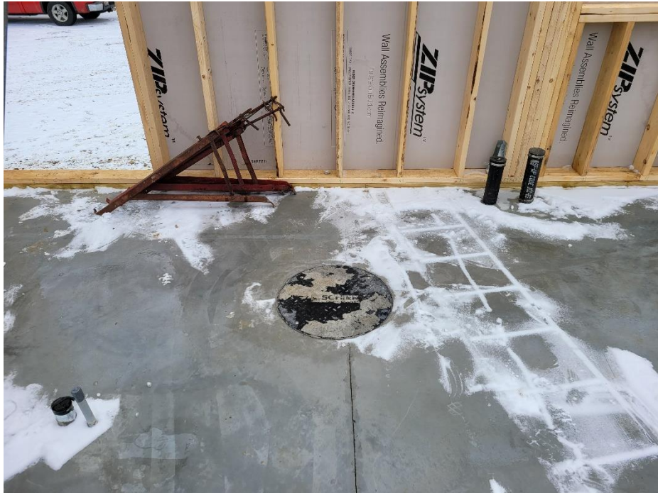
13. Grease trap cover at Kitchen
