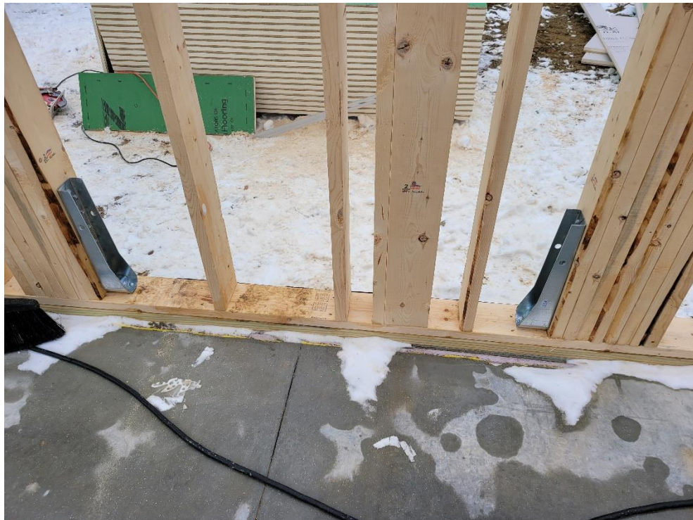
2. Detail of tie-downs at south wall of Office Wing
