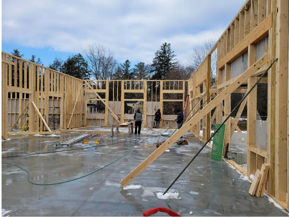
11. Classic carpenters installing blocking
