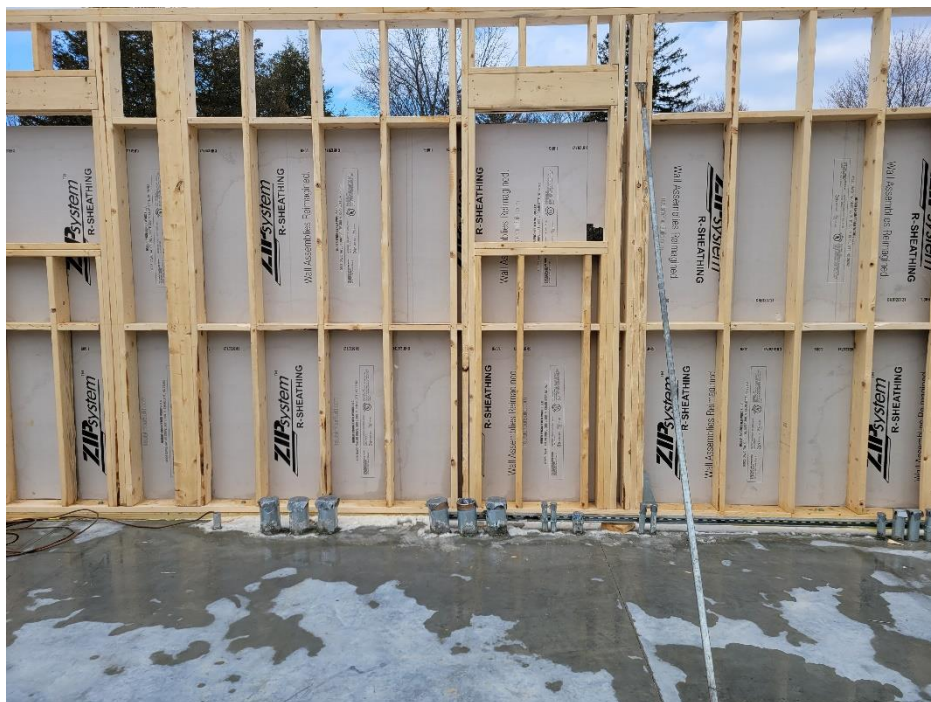
19. Parallam posts at interior wall to Multipurpose Room
