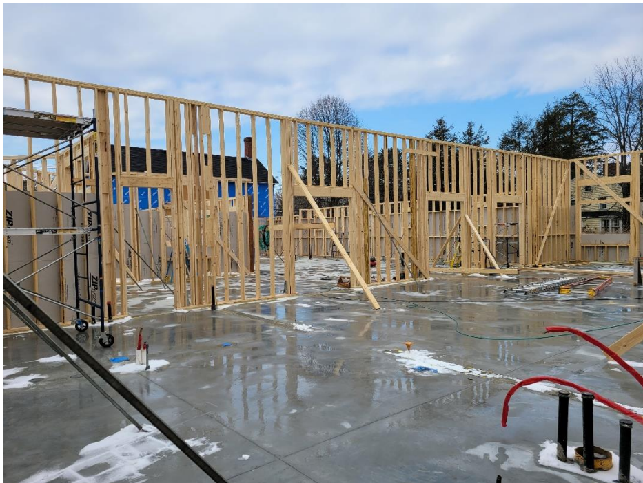
11. Classic carpenters installing blocking
