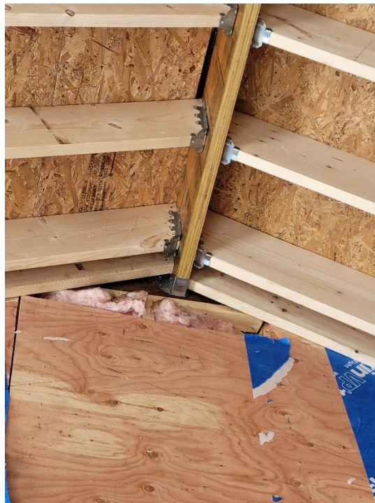
8. 14" deep LVL ridge beam at stick framed roof with connection to Cummings House
