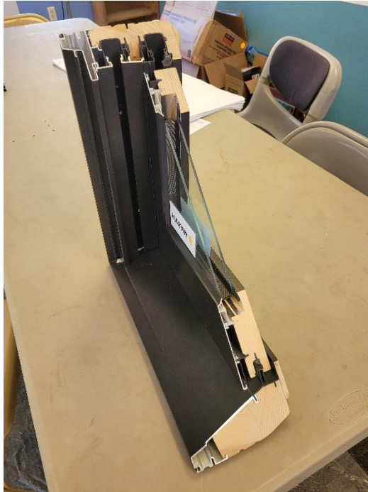
17. Sample cut of typical window at Addition- exterior aluminum cladding (sample only- final to be white)
