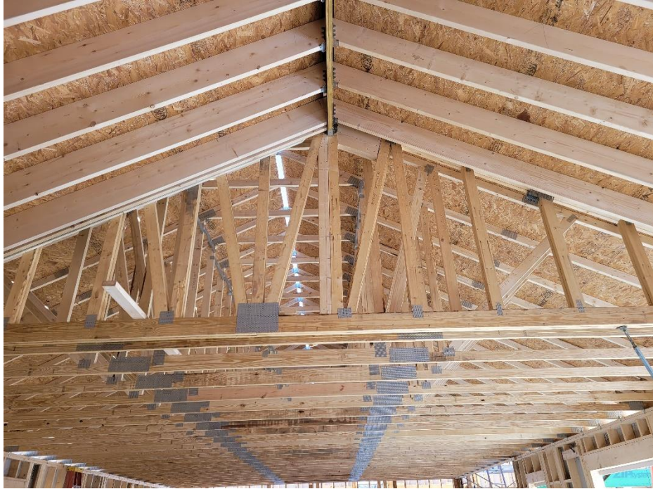
9. End truss at junction with stick framed roof
