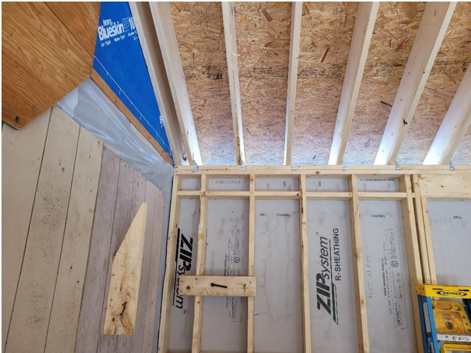
9. End truss at junction with stick framed roof
