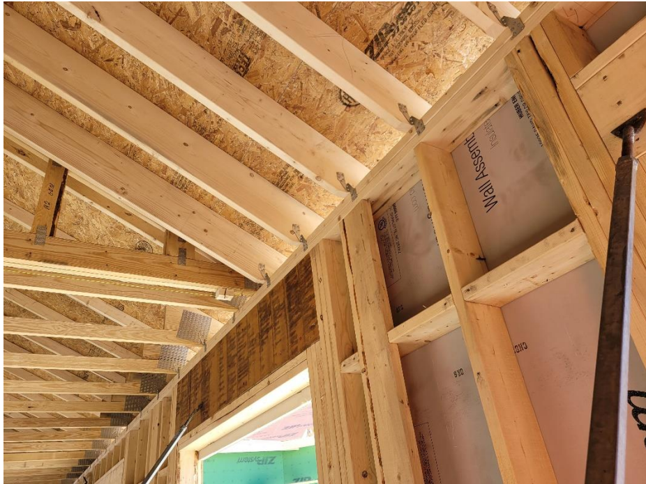
11. Rafter to plate connection at south wall
