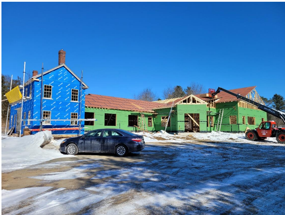
1. Roof sheathing installed on Office Wing and in progress on Multipurpose/ Kitchen Wing
