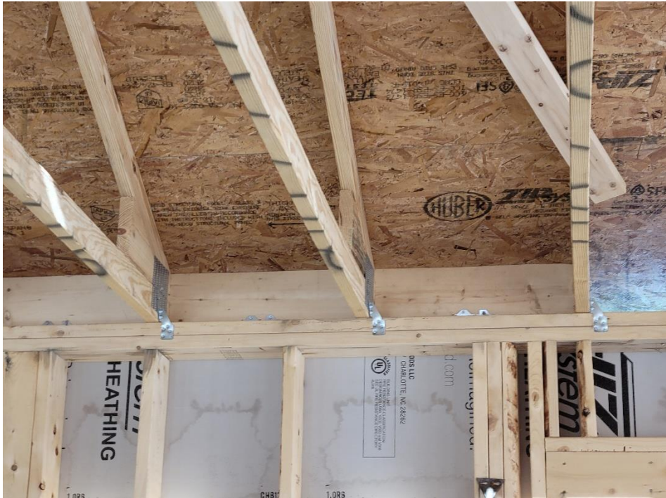
13. Shear blocking between trusses above shear wall (north wall)
