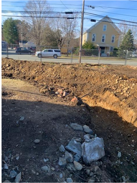
3. Trench for new water line to the well is excavated.
