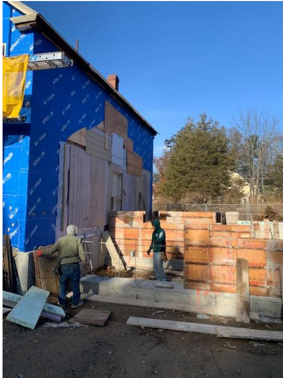
1. Formwork for final sections of foundation wall extending to East Wall of Cummings House being erected (view from south)
