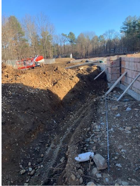
5. Trench excavation for new well water line extending to Addition at north site (Water Room location)
