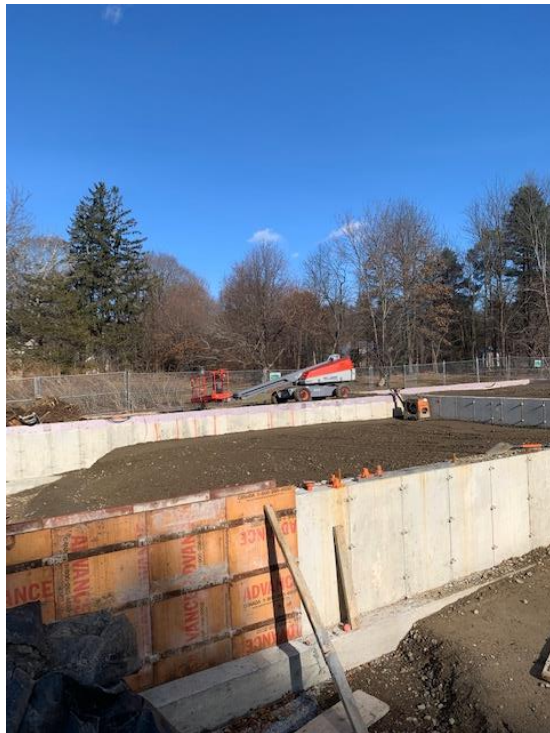
6. Fill material a new Addition installed and being compacted.
