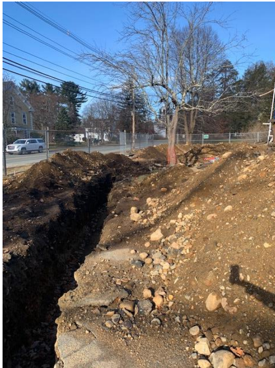
7. Water line trench along Elem Street
