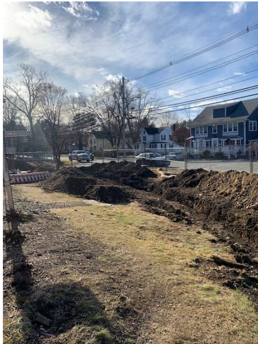
4. Trench for new water line to the well is excavated.
