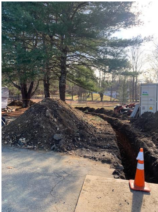
8. Well water line trench across driveway
