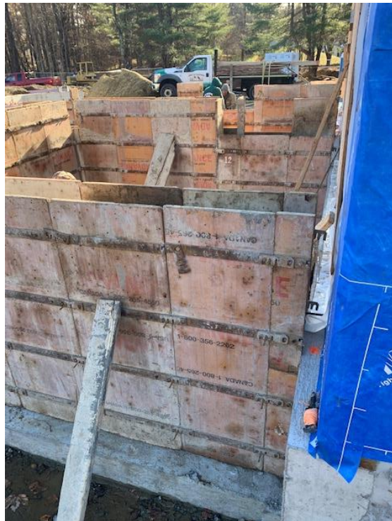
2 . Formwork for final sections of foundation wall extending to East Wall of Cummings House being erected (view from north)
