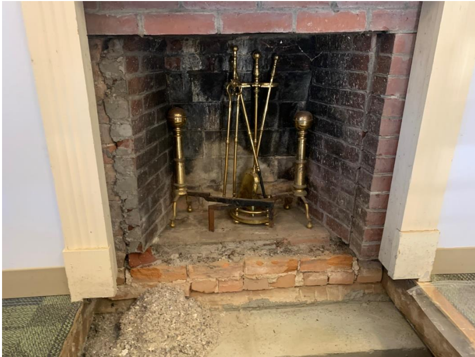
11. North firebox at Cummings house; hearth being prepared for new brick hearth finish.
