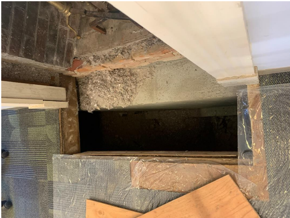
11. North firebox at Cummings house; hearth being prepared for new brick hearth finish.
