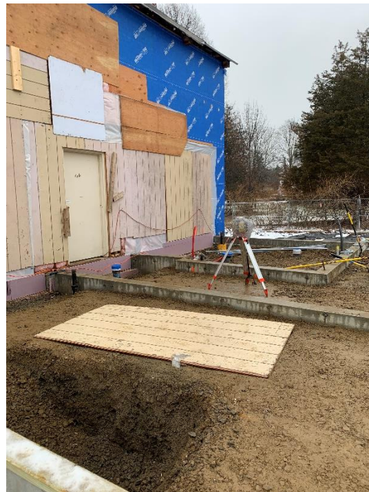
4. New Addition foundation and backfill completed.
