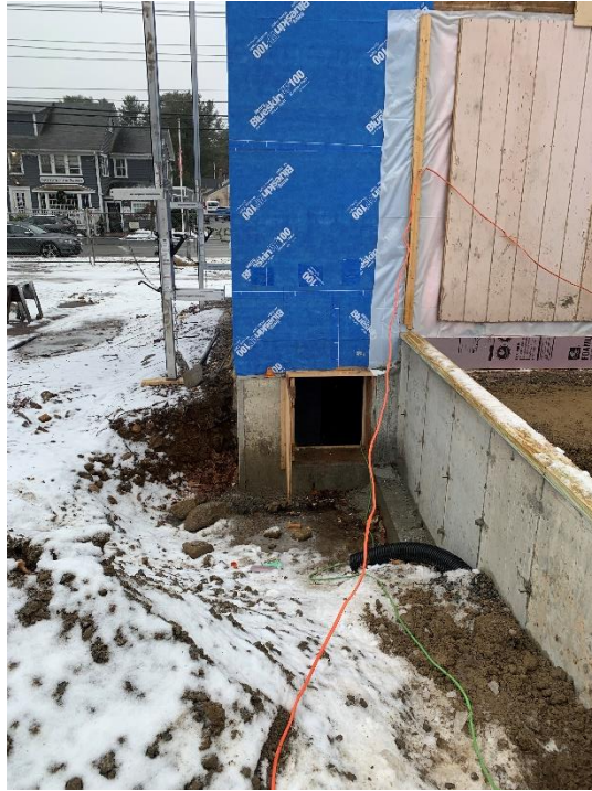
3. Opening for Turtl Access hatch at southeast corner of Cummings Basement/ crawlspace.
