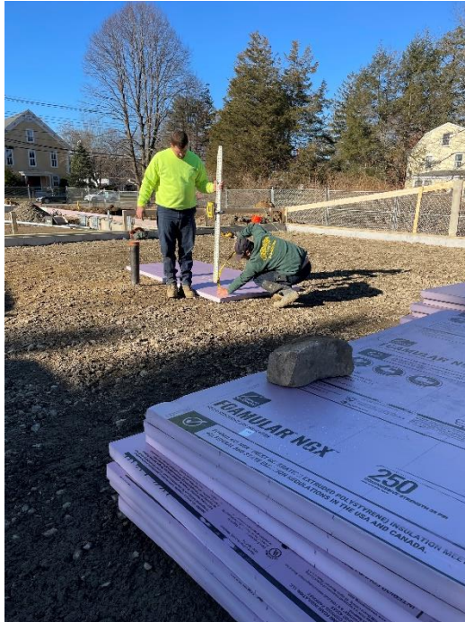
9. Verification of top of insulation elevation to ensure 4" min. slab thickness (photo by Fred Scibelli 12/17/21)
