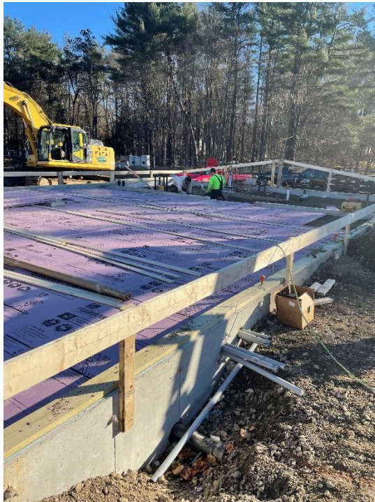
7. Preparation of Multipurpose/ Kitchen slab with rigid insulation and wood framing for heating tent (photo by Fred Scibelli 12/17/21)
