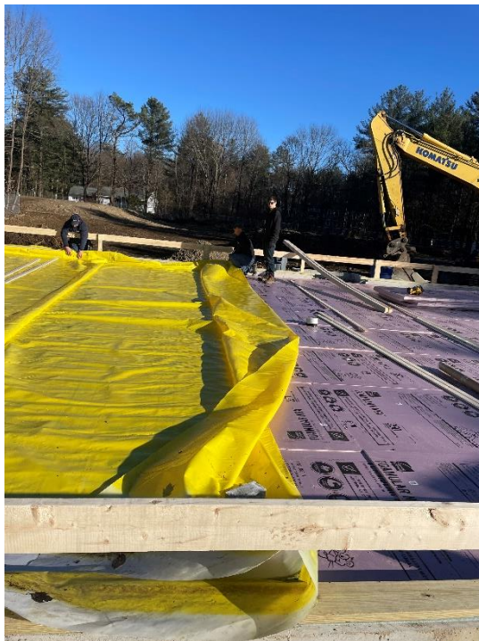
7. Preparation of Multipurpose/ Kitchen slab with rigid insulation and wood framing for heating tent (photo by Fred Scibelli 12/17/21)
