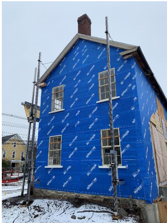
2 . Air barrier (Henry Blueskin VP-100) installed completely on South, West and North sides of Cummings House.
