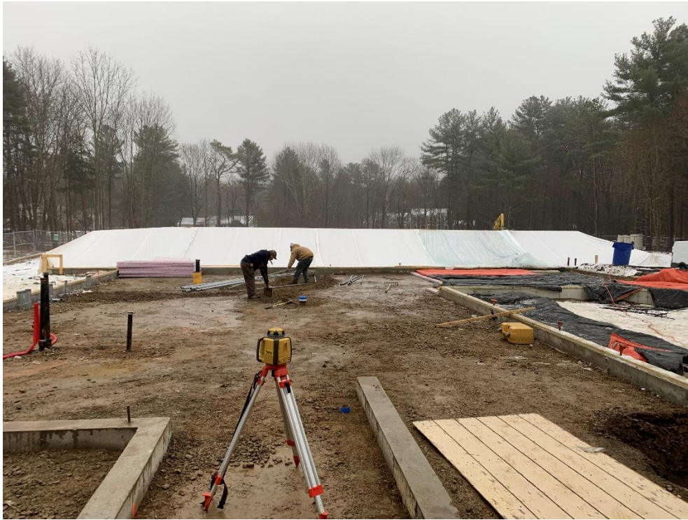
1. Slab poured at Multipurpose/ Kitchen Wing on 12/21/2021, tented and heated during the 7-day wet-cure; Office wing slab to follow next week.
