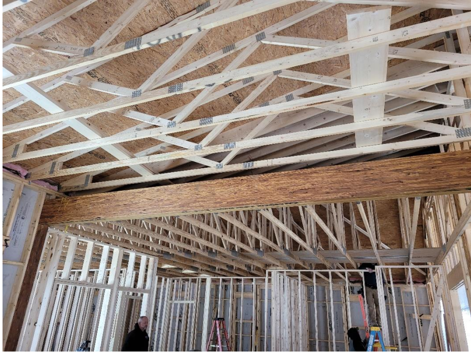
11. Truss framing above Lobby at dropped beam
