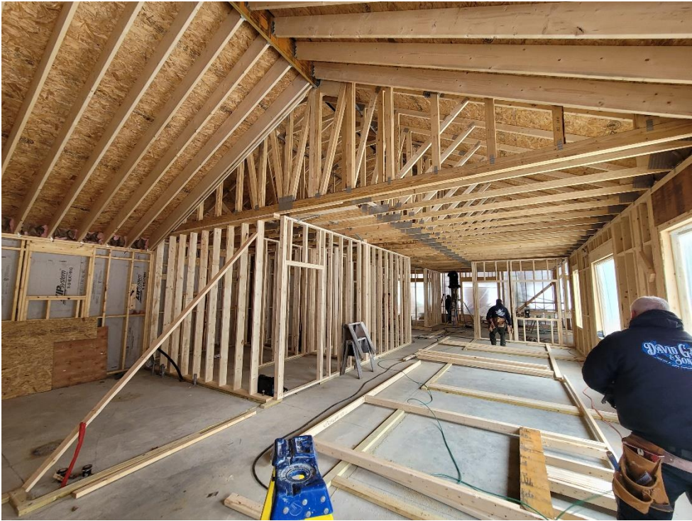
5. Stick-framed roof above Water Room (foreground left)
