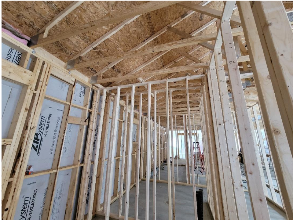
7. Wall framing at underside of trusses (Men's Room)
