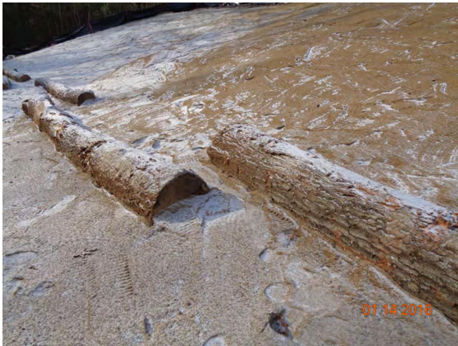
Photograph 10: View of reclaimed snags embedded in slope for stability.
