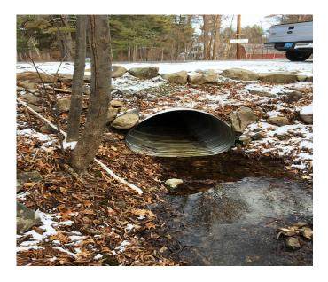
The Topsfield Road drainage pipe is shown above. It is located near the intersection with Pinehurst Road. The new pipe was installed in August 2016 during a one day shutdown of Topsfield Road. The DPW continues to replace deteriorated drainage pipes throughout the Town in accordance with a schedule 5 years ago via an engineering study of the Townøs drainage systems.
